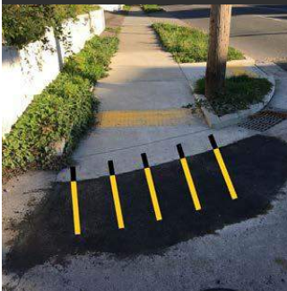
Correct Placement of Smart Level for Measuring Running Slope of New Asphalt Connection
