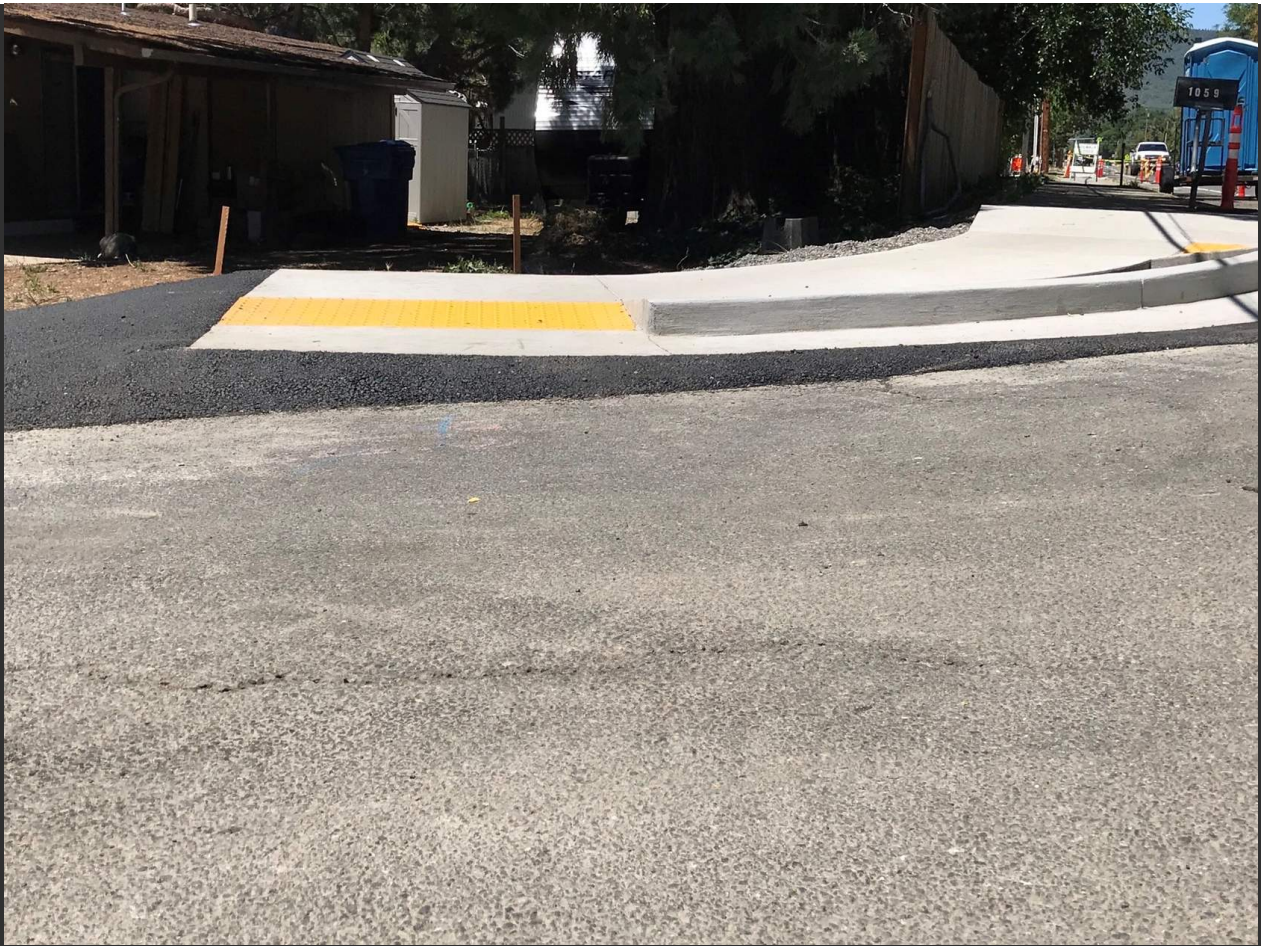
A non-compliant asphalt connection
