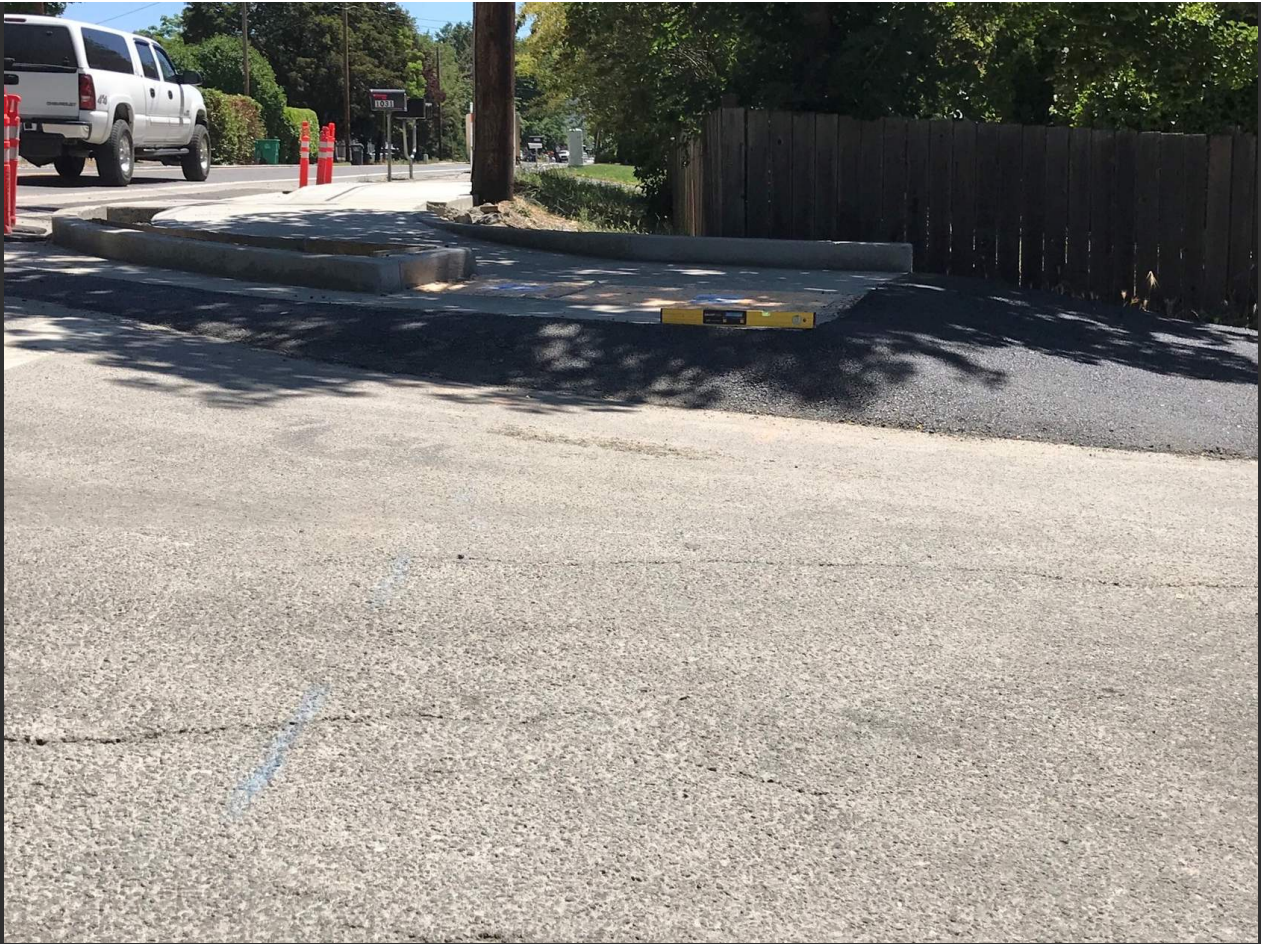
A non-compliant asphalt connection
