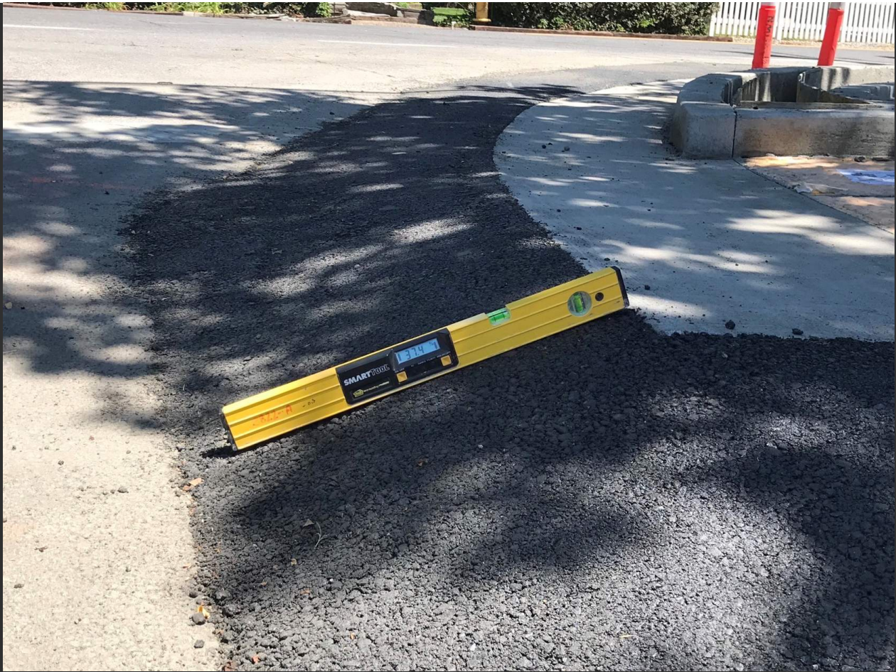
A non-compliant asphalt connection
