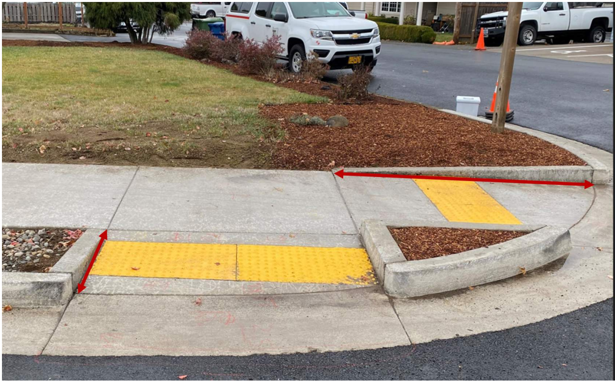
Curb Ramp System with Dimension Lines for Ramp Run Lengths.
