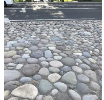
Grouted Durable Rock Example 4
