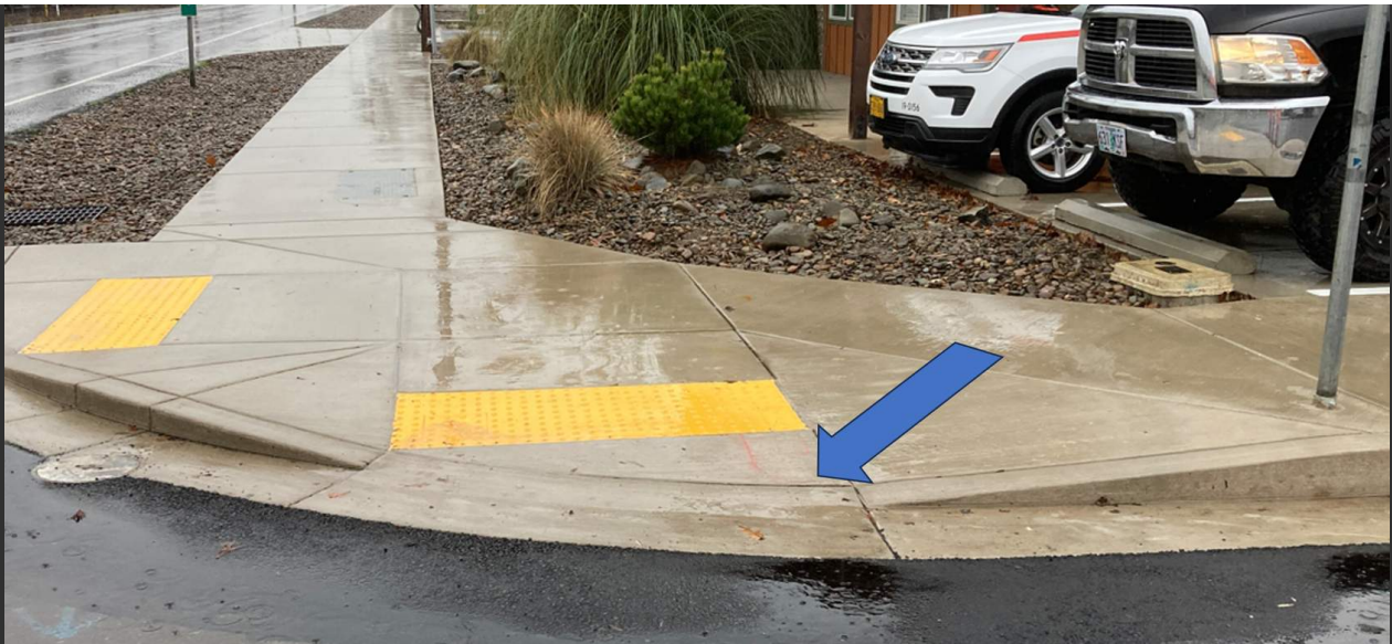
Improperly Installed Detectable Warning Surface. Pedestrian with Visual Impairments Could Miss Detectable Warning
