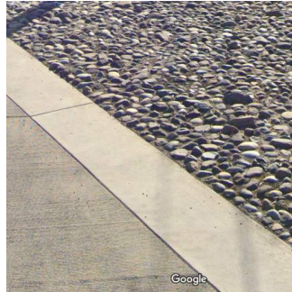
Grouted Durable Rock Example 2
