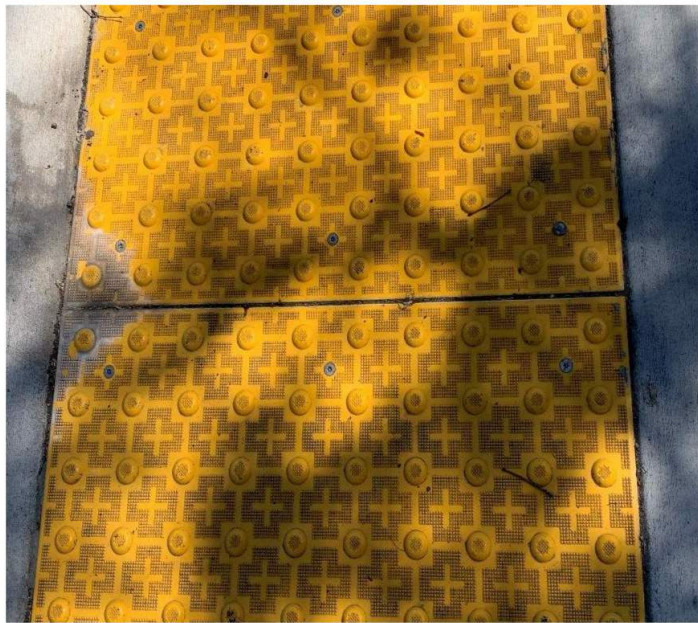
Correct Installation of Adjacent Panels
