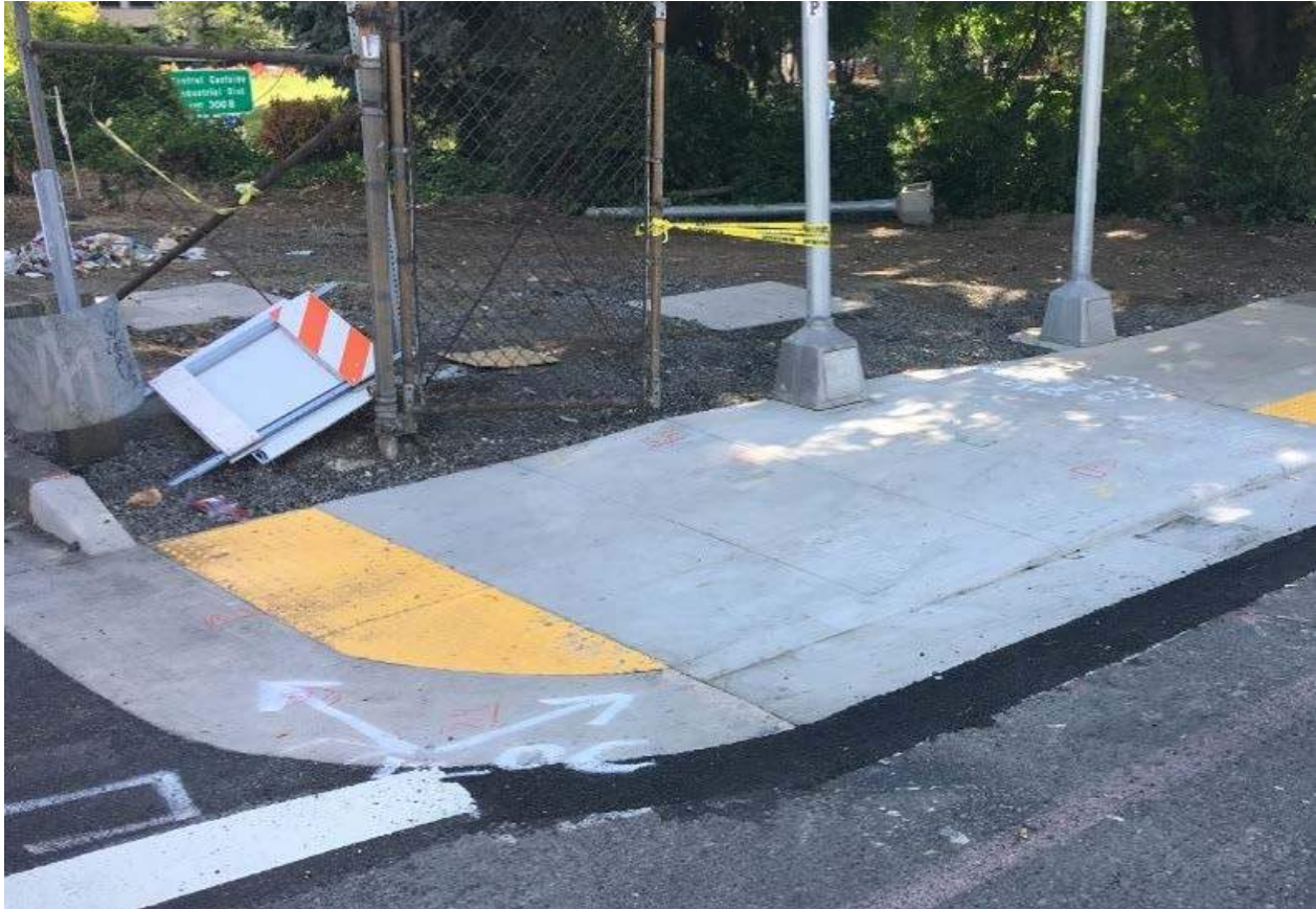
Improper Detectable Warning Surface Cut To fit The Radius of The Curb
