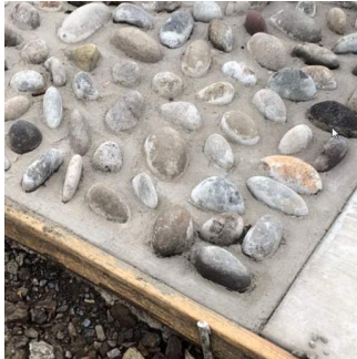
Grouted Durable Rock Example 1
