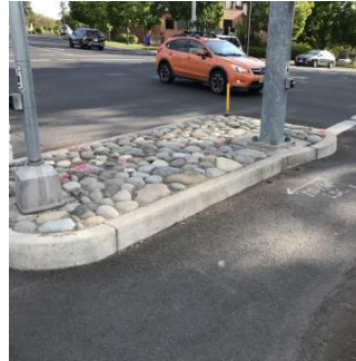
Grouted Durable Rock Example 3
