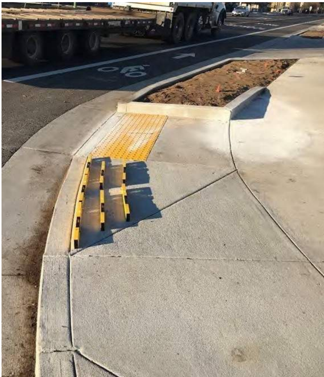
How to Place Smart Levels on a Flare
