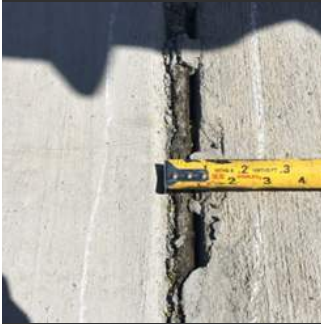
Expansion Joint Gap Failures
