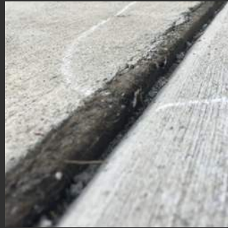
Expansion Joint Lip Failures
