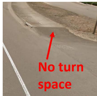
End of Walk Curb Ramp that Does Not Require a Turn Space
