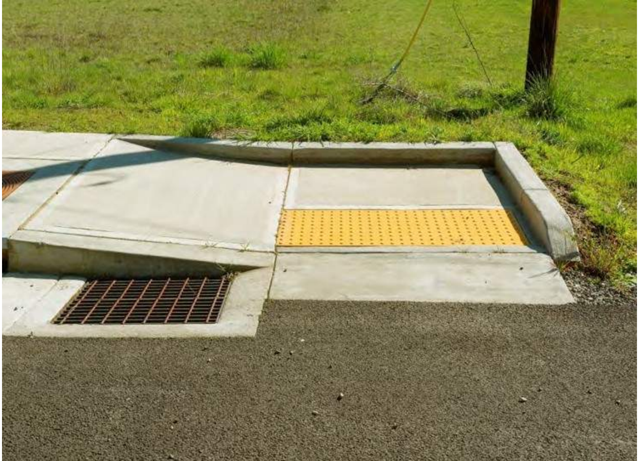
A One-Sided Parallel Ramp is Considered a Unique Design Style Curb Ramp
