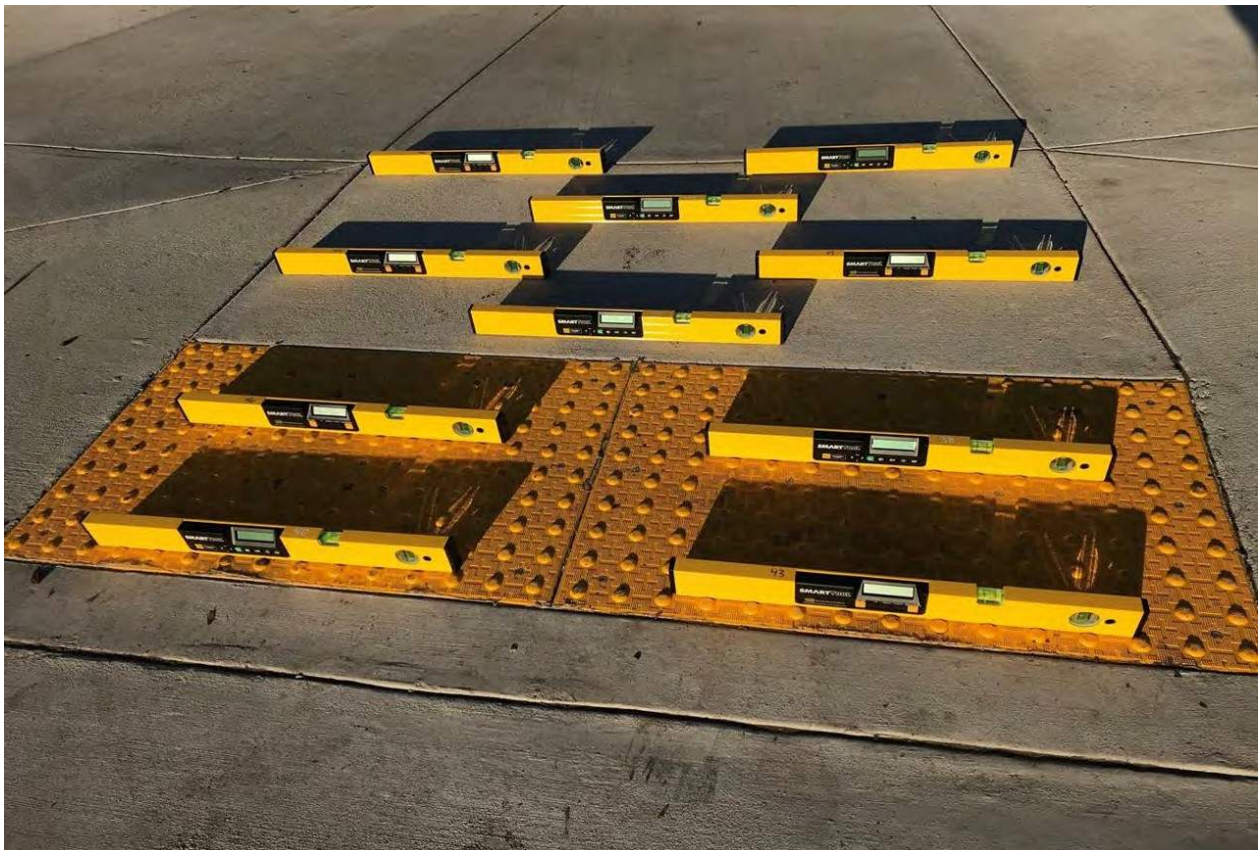
Example of how to Measure Cross Slope on a Perpendicular Curb Ramp System
