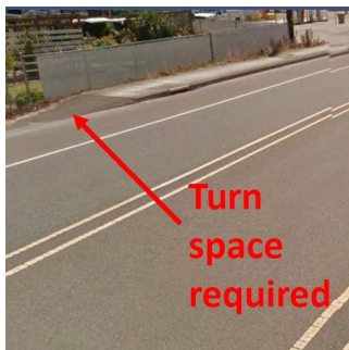
End of Walk Curb Ramp that Requires a Turn Space for
