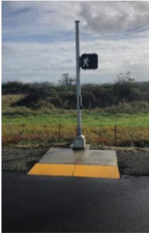
Concrete Pedestrian Pad to Access Pushbutton at a Signalized Intersection
