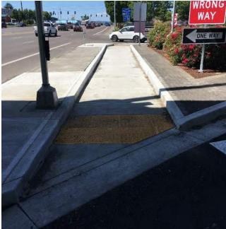
A Cut Through with a through movement that may or may not require a Turn Space depending on Running Slopes
