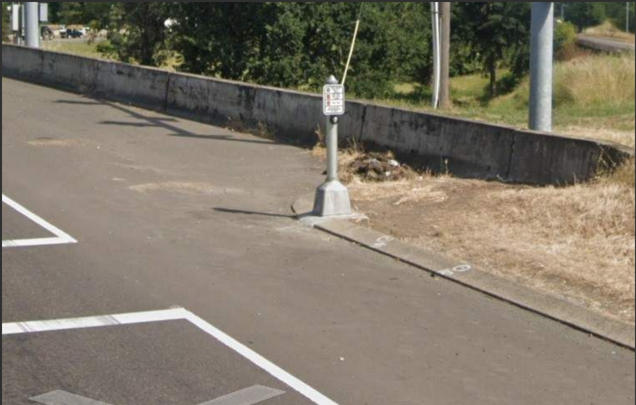
Paved Shoulder Pushbutton Clear Space, No Curb Ramp System Constructed
