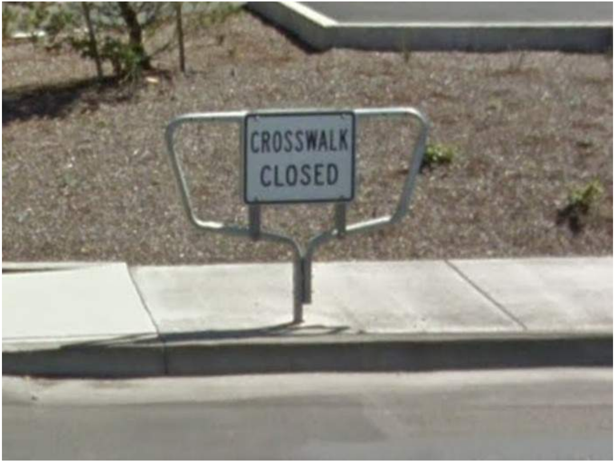
Proper installation of a Crosswalk Closure Support
