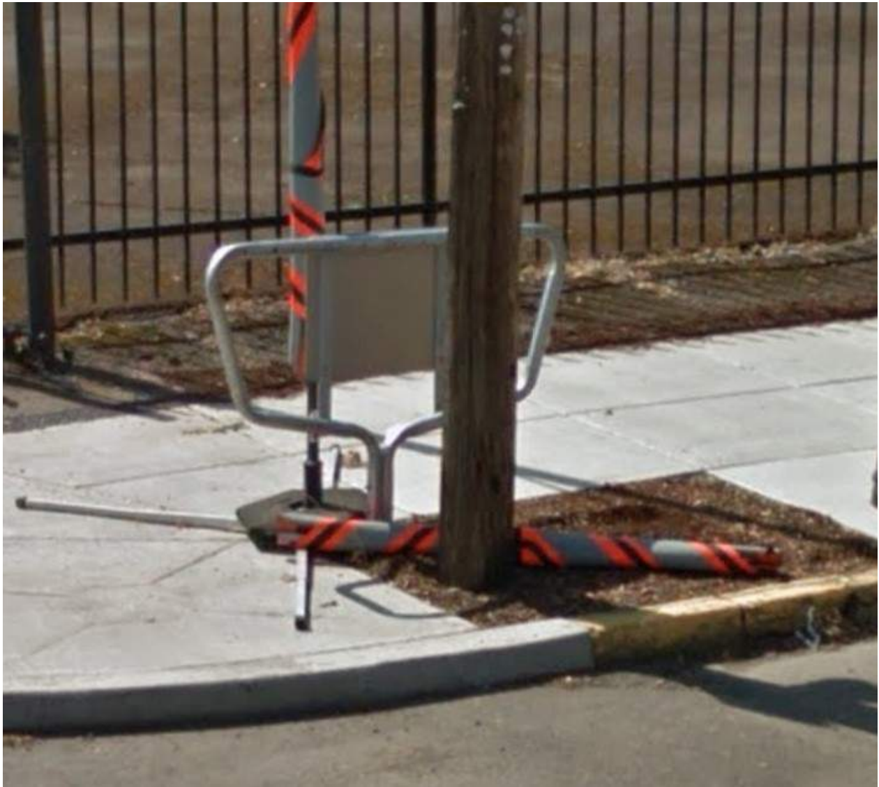
Example 2: of Incorrectly installed crosswalk closure support
