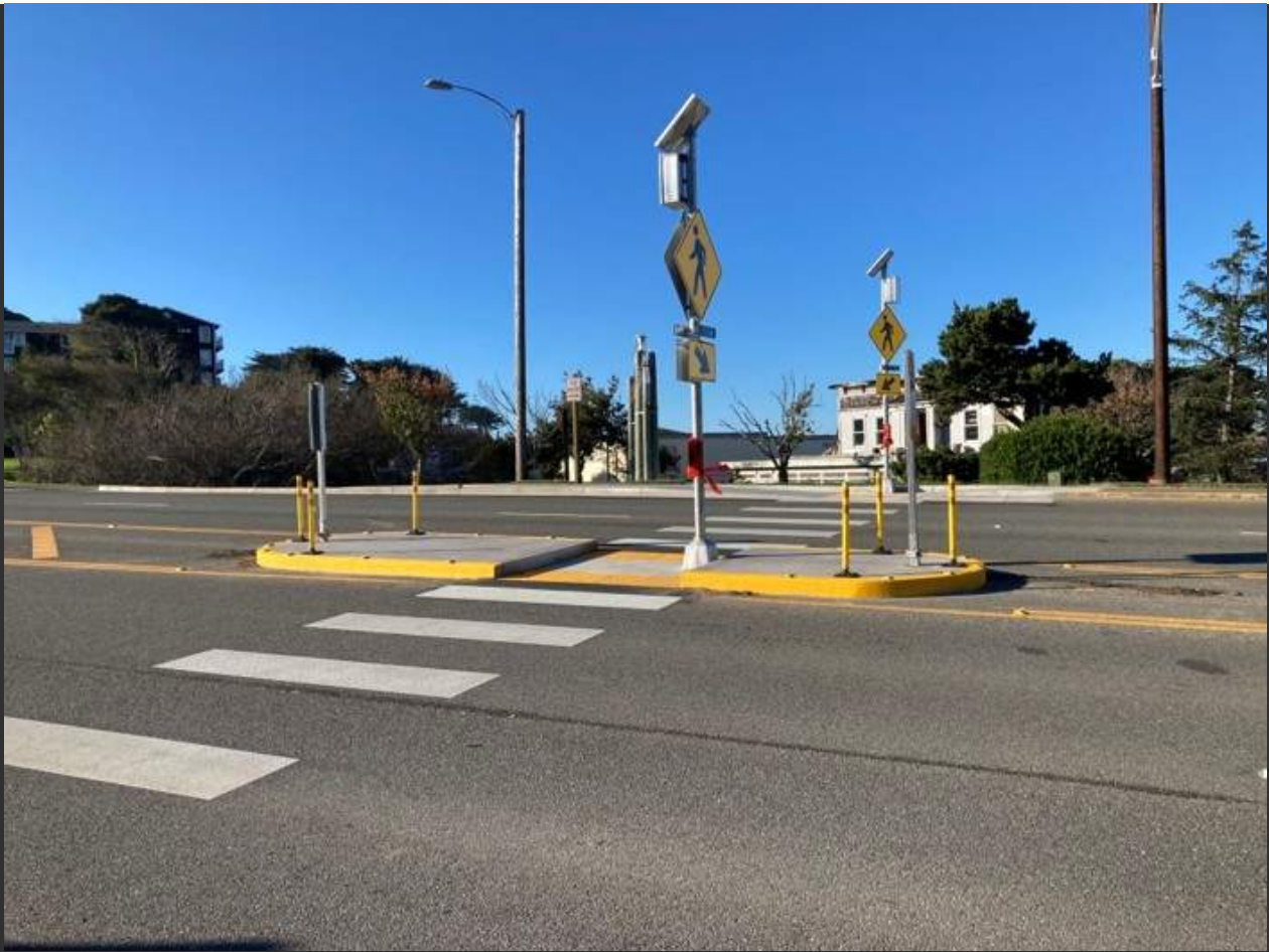
Pedestrian Island with continuous yellow curb adjacent to yellow detectable warning surface (truncated domes) does not provide contrast.
