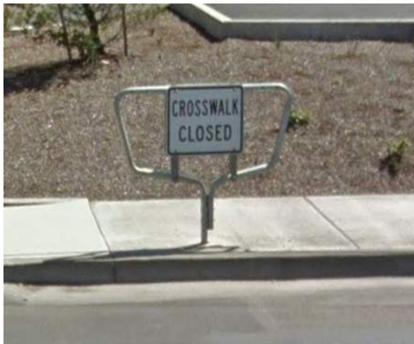
Proper installation of a Crosswalk Closure Support
