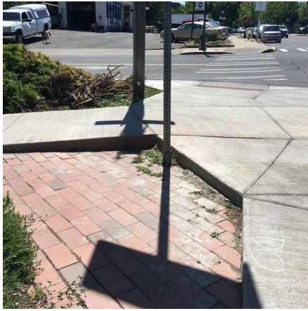
Drop Off Photo 1: Vertical discontinuities within curb ramp proximity limits will result in failure.
