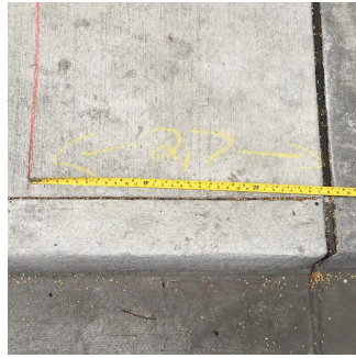
5.0 feet Between Ramp Runs Photo 2- 2:
