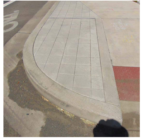
Drop Off Photo 3: Curb Ramp designs that include a buffer strip must use a non-walkable surface. Concrete, stamped/colored concrete, or pavers will result in failure.
