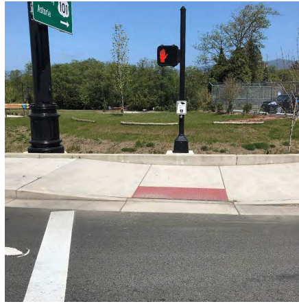
F/W issues Photo 2-1: A newly constructed parallel ramp with isolated slope issues on the turn space.
