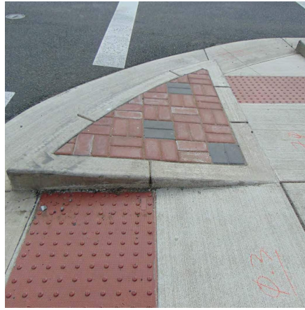
Drop Off photo 2: Curb Ramp designs that use return curb creating a triangle piece between the two ramp positions requires a non-walkable surface to be installed.
