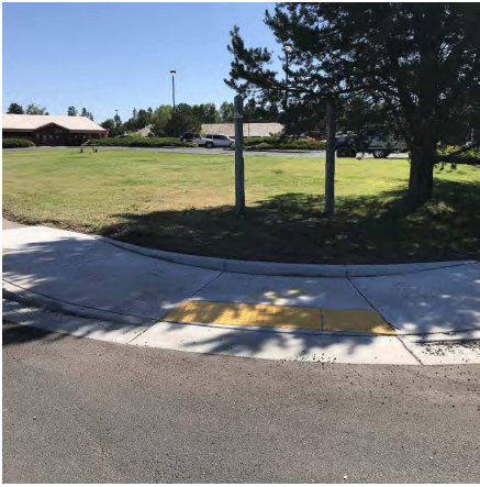
F/W issues Photo 1: A newly constructed parallel ramp with a ramp run 3 that is crumbling at the curb.
