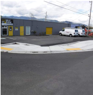
5.0 feet Between Ramp Runs Photo 1-1: Two combination style ramps that do not meet the 5.0' between ramp runs requirement.
