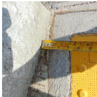
Truncated Domes Photo 4: Truncated domes are required to be within 2.0 inches on both
