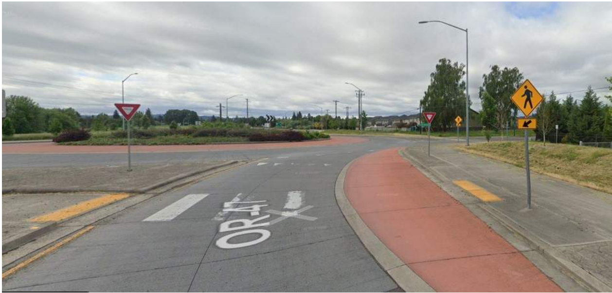
Truck Apron at a Roundabout
