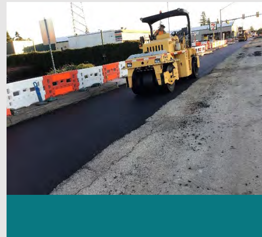
Pneumatic Roller used
