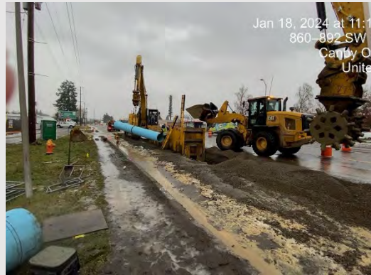
Mainline Pipe Work
