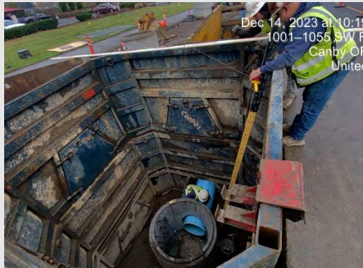
Drywell Installation
