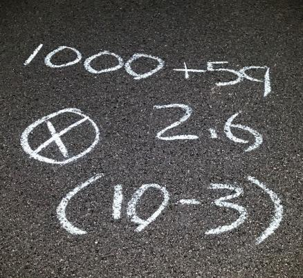
\* Site Locations must be marked after finish rolling, S ASAP, to prevent Construction delays.
