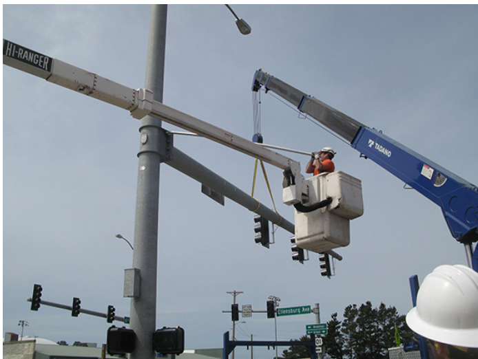
Bolt Tightening with Cheater Bar (May be difficult to achieve proper tensioning)
