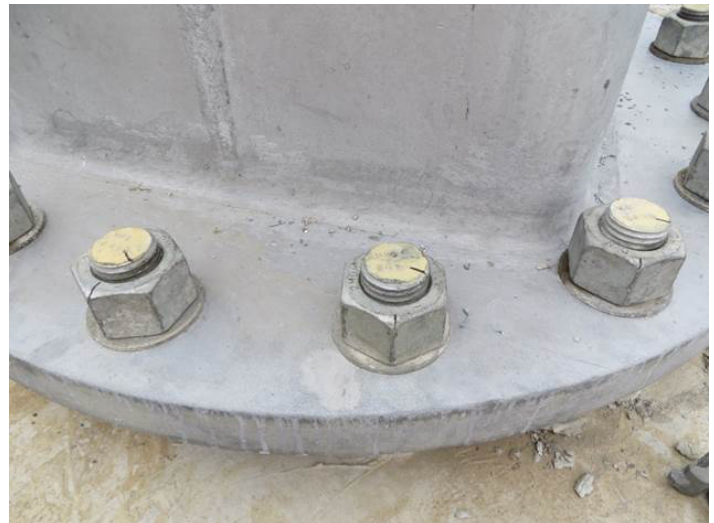
Tightened Bolts Photo shown for illustration of bolt markings only. Signal anchor bolts require two nuts per bolt.
