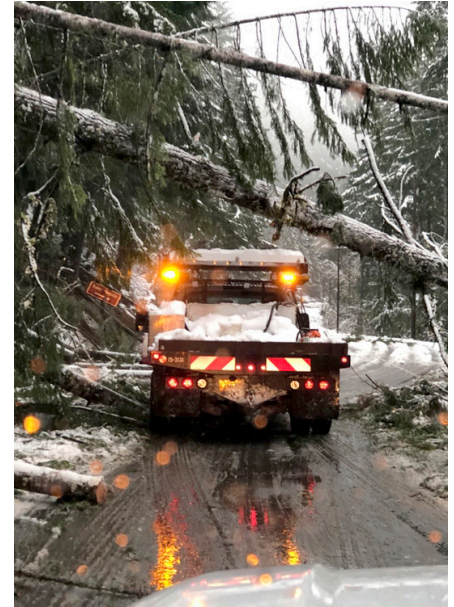
Maintenance crews work to remove fallen trees on OR 138E.
