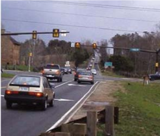
Intersection where the traffic signals were converted from a night-time flash mode to a normal steady operation
