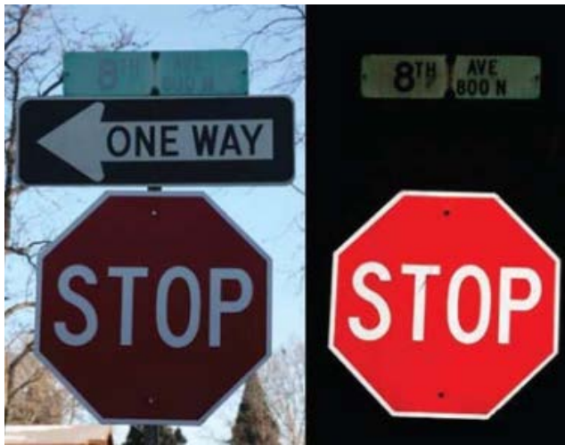
Retroreflective stop sign in daylight and nighttime conditions Image from FHWA
