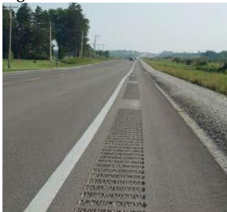
Figure 6-18. Shoulder Rumble Strip
