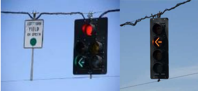
Figure 4-8. Doghouse Signal and Flashing Yellow Arrow
