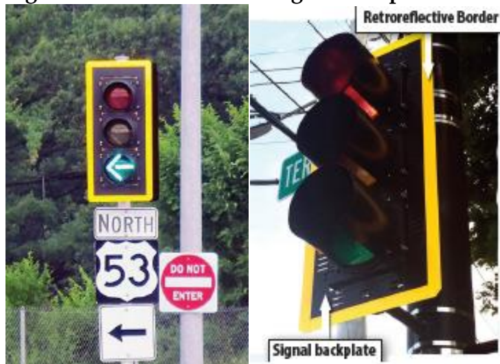
Figure 4-3. Retroreflective Signal Backplate
