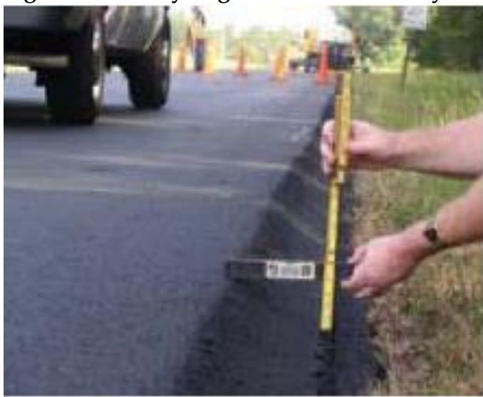
Figure 6-5. Safety Edge for Rural Roadway
