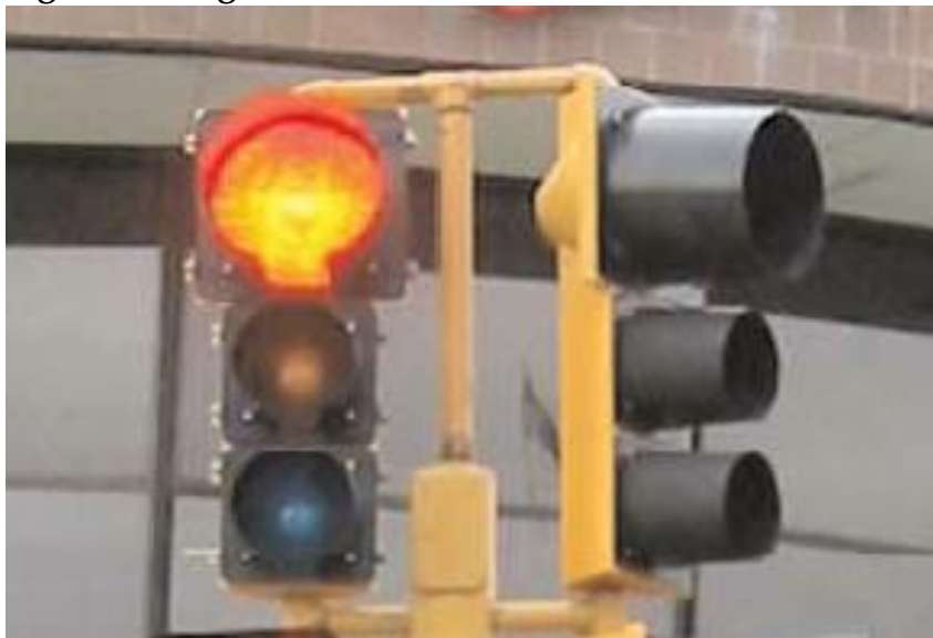
Figure 4-4. Signal Heads with 8-inch and 12-inch Lens
