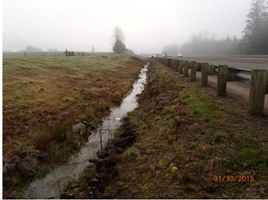
example of photo 5 upstream roadside channel that drains into stormwater facility
