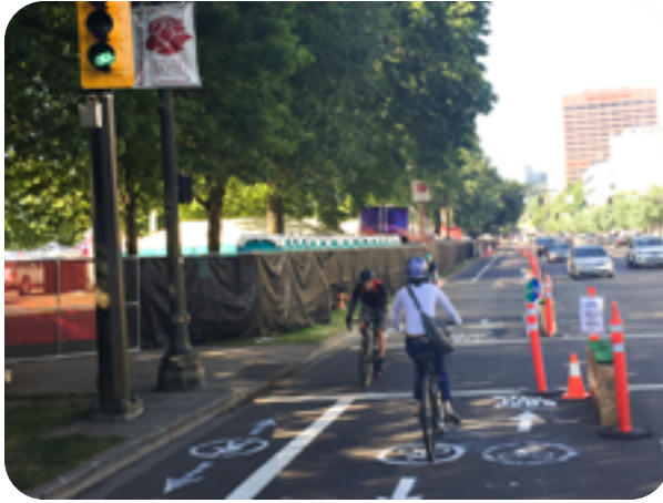
Quick build project in Portland using temporary barriers and pavement marking to create a multiuse path in the roadway, which was later turned into a permanent multiuse path. Photo from Metro.
