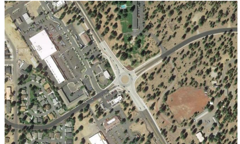
Example of a recommended and implemented countermeasure
