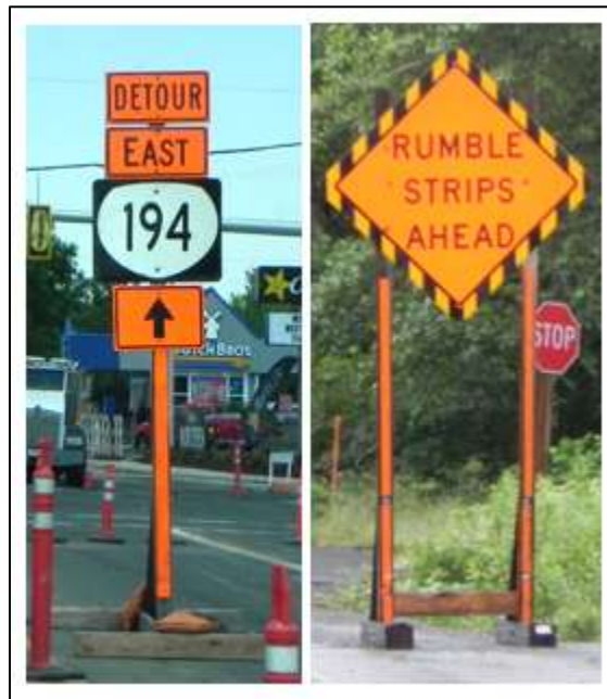
Figure 2-14: Temporary Sign Supports
