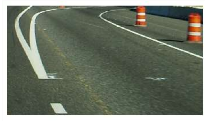
Figure 2-4: Temporary Striping for Exit Ramp
