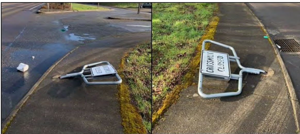
Figure 310.8-1: Damaged Crosswalk Closure Treatment
