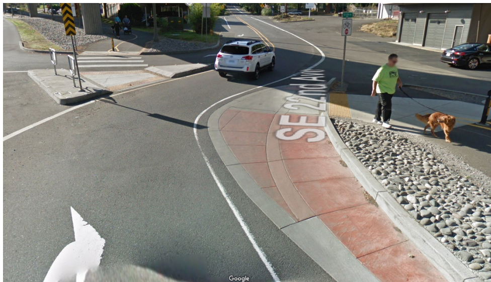
Exhibit 500-1: Apron to Accommodate Bus Turning and Minimize Radius for Passenger Vehicles
