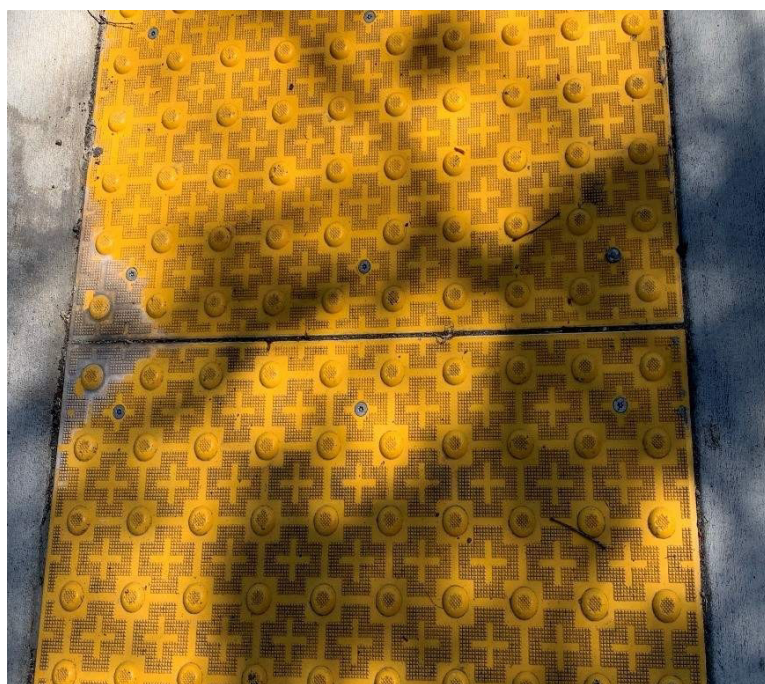
Figure 800-59: Wet Set Polymer Detectable Warning Surface Tile Dome Spacing is Maintained
