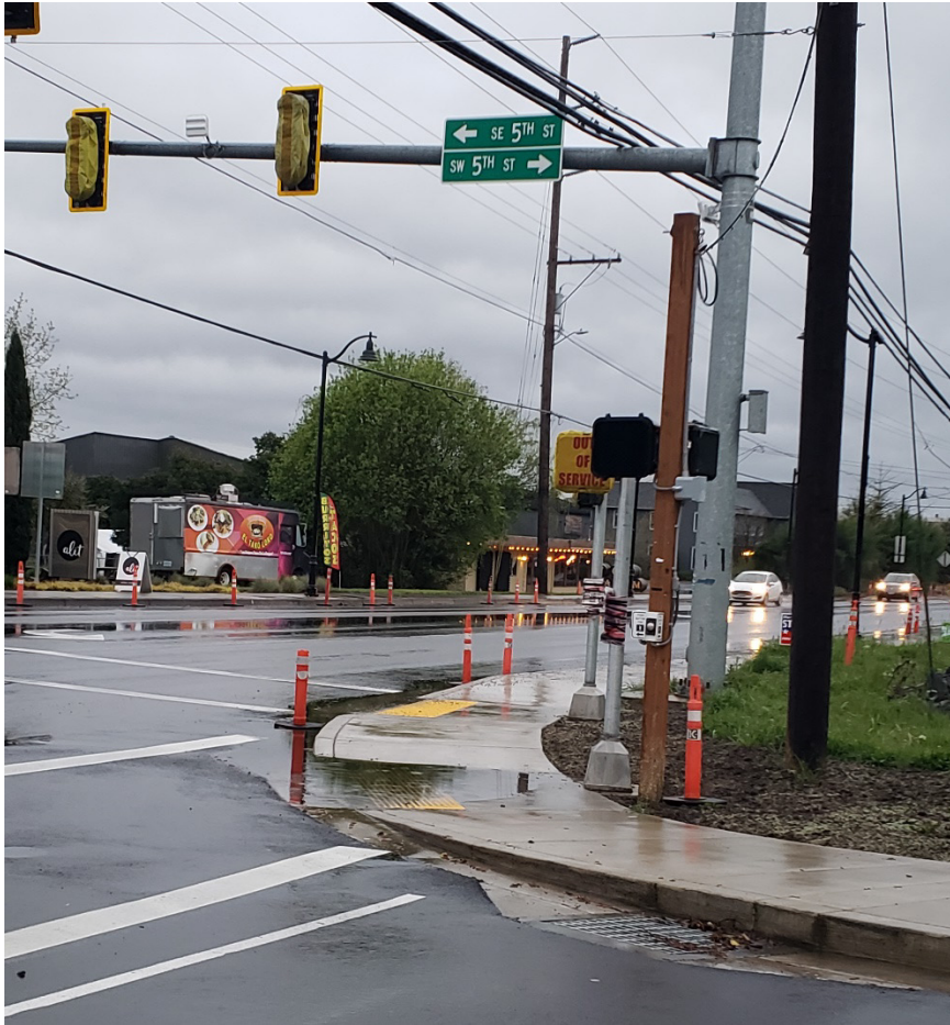
Figure 800-44: Water Accumulation at Curb Ramp
