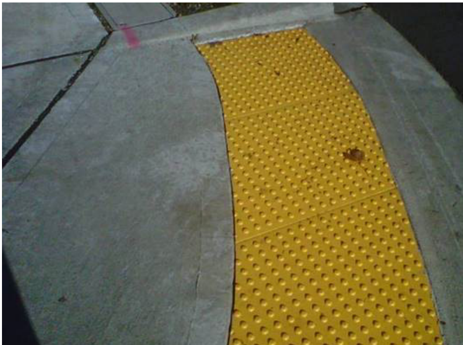
Figure 800-64: Example 2, Detectable Warning Surface Rectangular Tile Cutting to Fit Radius
