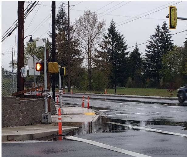
Figure 800-52: Water Accumulation at Curb Ramp on Landing/Turn Space
