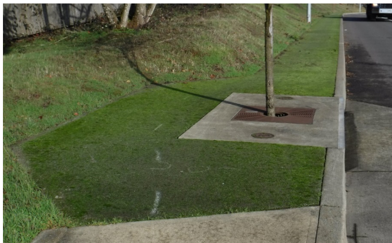
Figure 800-22: Porous Pavement Installed Next to Concrete Walk Illustrating Mossy Growth
