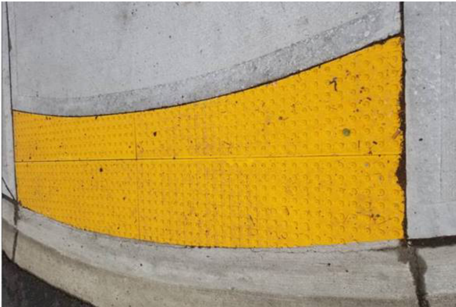
Figure 800-64: Example 2, Detectable Warning Surface Rectangular Tile Cutting to Fit Radius
