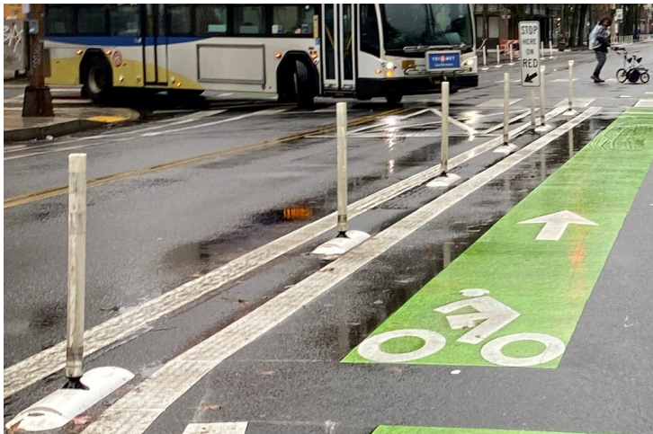
Figure 900-12: Tubular markers as street buffer
