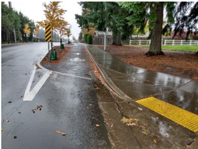
Figure 900-11: Landscape Buffer Cross Section at Street Crossing
