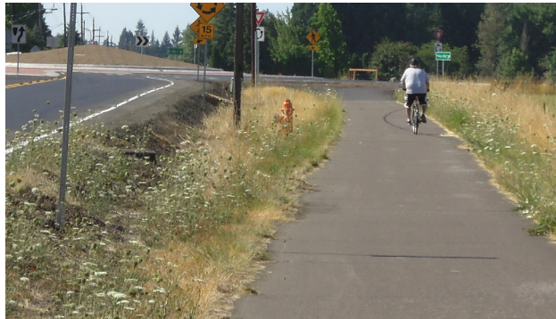
Figure 900-16: Roadside ditch as street buffer
