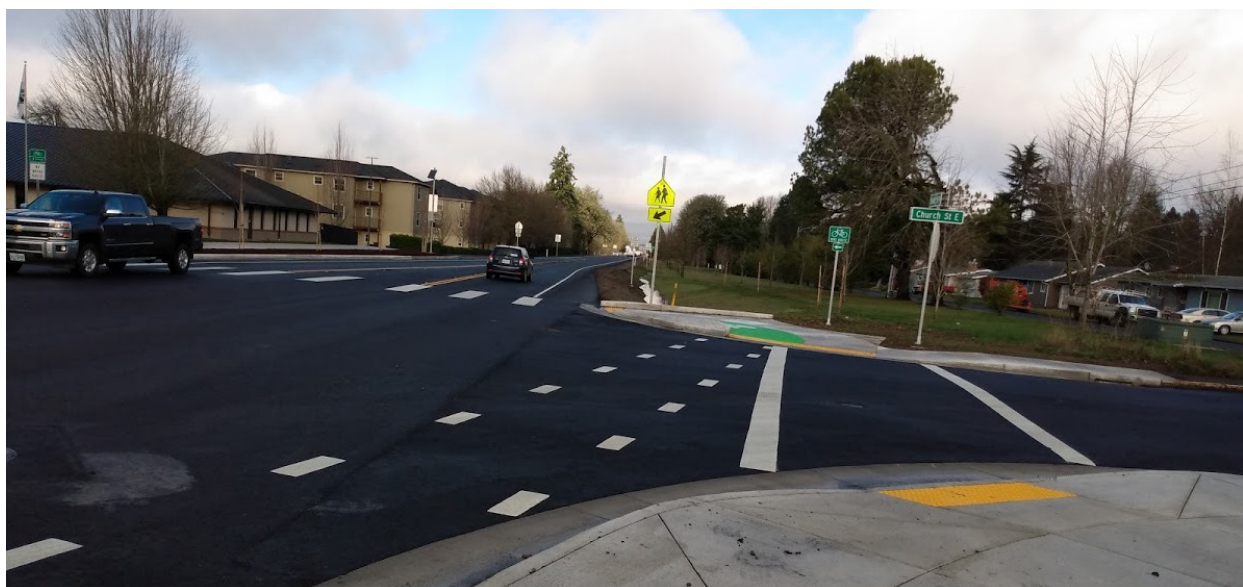
Figure 900-18: Transition from bike lanes to side path across street uses corner to position bicycles at crosswalk.
