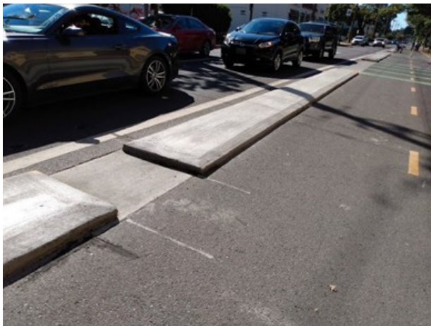
Figure 900-10: Island Buffer Cross Section with Drainage Gap
