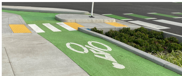
Figure 900-17: Bio-swale as street buffer
