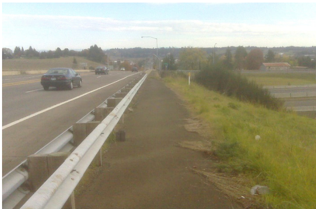
Figure 900-15: Guardrail in street buffer
