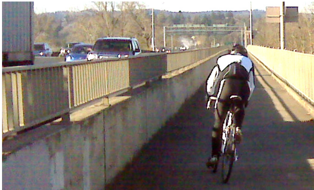
Figure 900-14: Concrete barrier as street buffer
