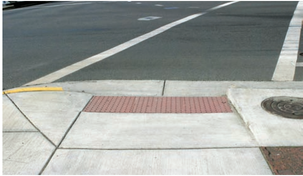
Curb ramp with one flare
