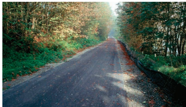
Gravel shoulders prevent raveling of path edges
