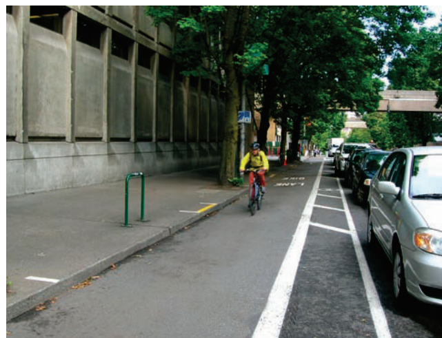
Parallel parking lane as street buffer
