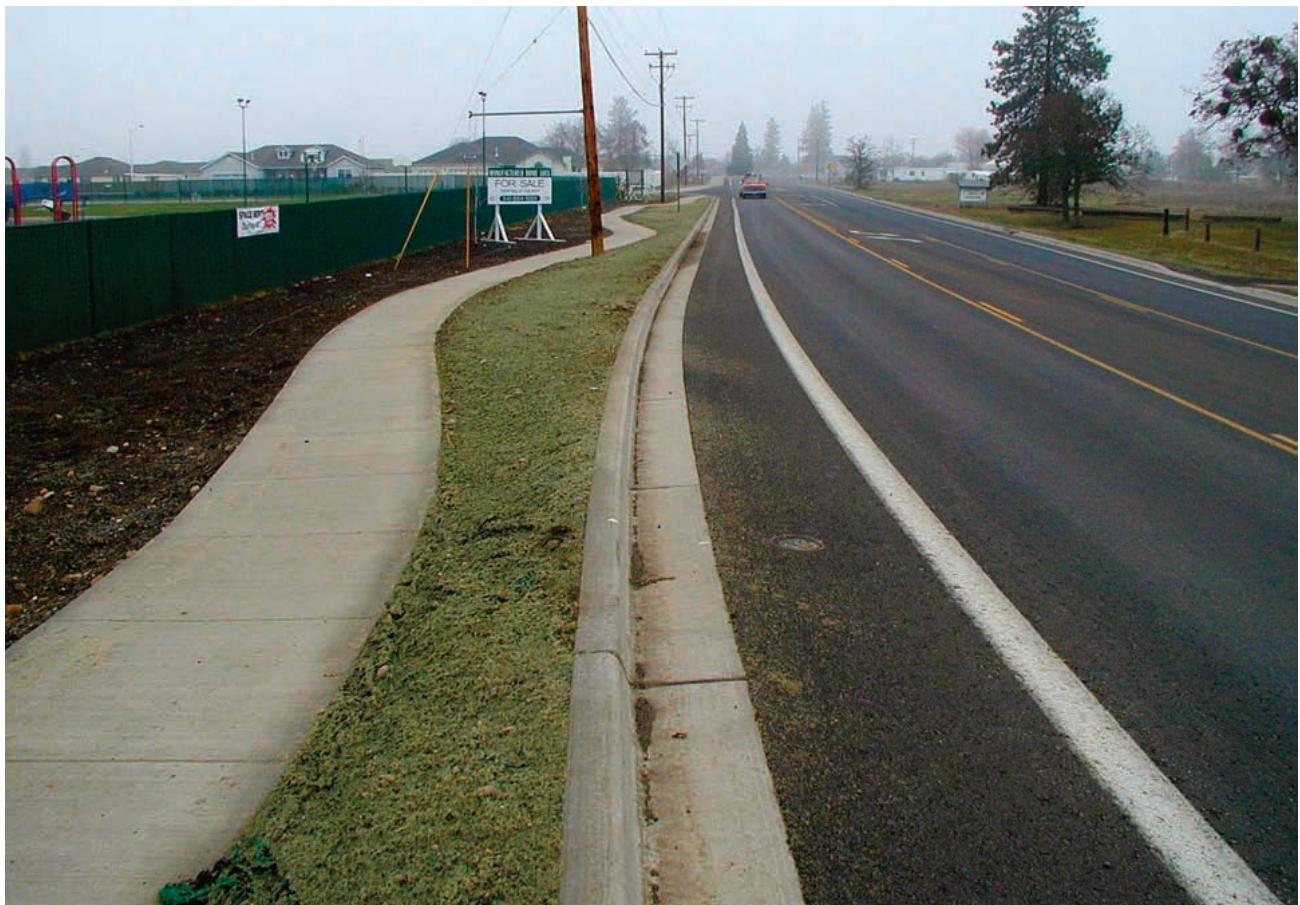
Meandering a sidewalk for no purpose should be avoided.
