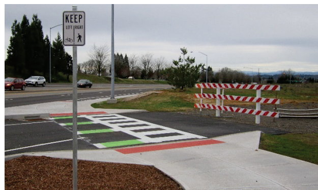
Detectable warning surfaces extend across entire path –pedestrian and bicycle zones.
