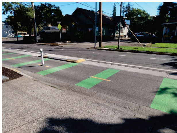
Figure 1-23: Pavement markings to highlight conflict point at driveways along bi-directional bike lane
