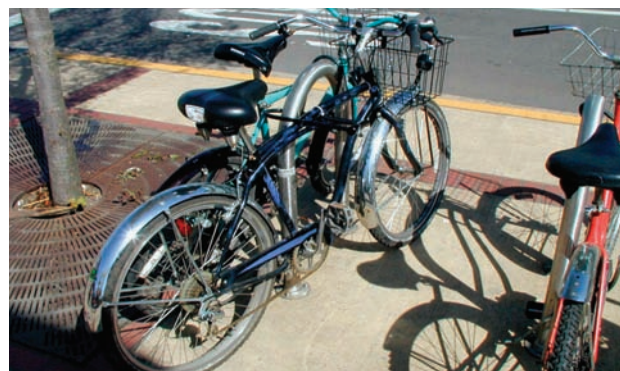
Upside down U or staple rack accommodates two bicycles
