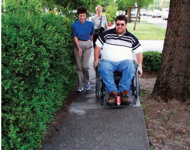
5 foot sidewalk is uncomfortably narrow
