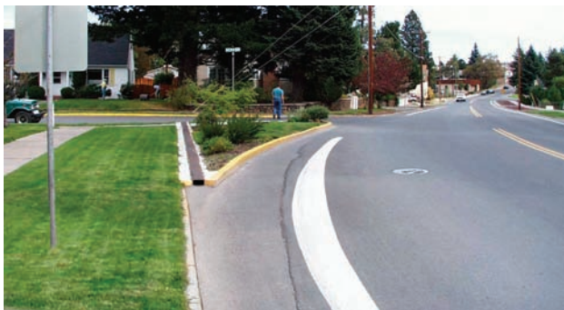
Formerly skewed intersection realigned to right-angle
