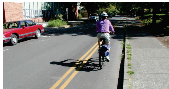
Contra-flow bike lane: One way for cars, two way for bicycles
