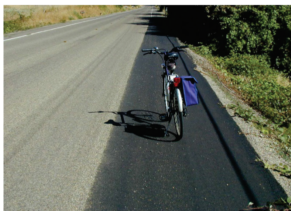
Chip seal ends at motor vehicle travel lane
