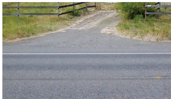
Paved driveway apron keeps gravel off shoulder
