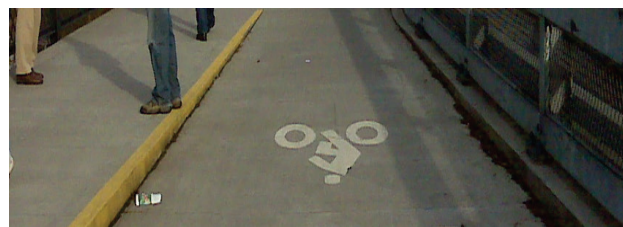
Bridge with curb between bike lane and sidewalk, indicating that users are not intended to mix.
