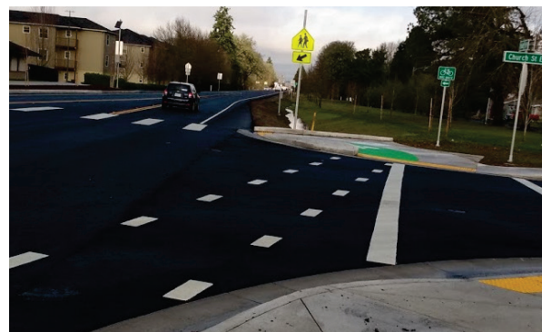
Figure 1-24: Transition from bike lanes to side path across street uses corner to position bicycles at crosswalk.
