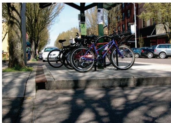
Slotted drain at retrofit curb extension
