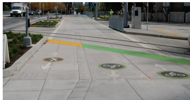
Pavement markings indicate which side of path each user is expected to use.
