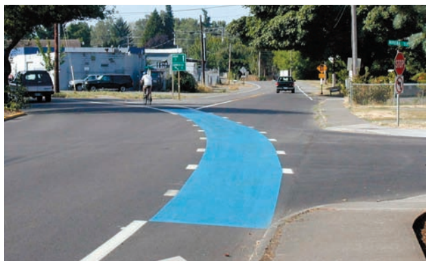
Blue bike lane thru skewed intersection
