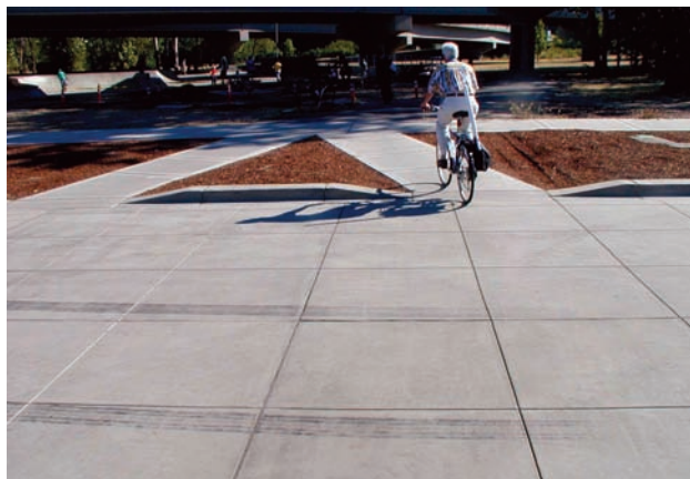
Split path entry eliminates need for bollards
