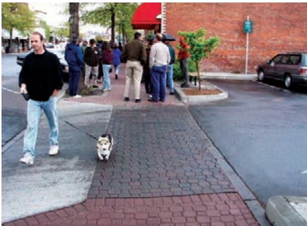
Sidewalk thru alley entrance is kept level
