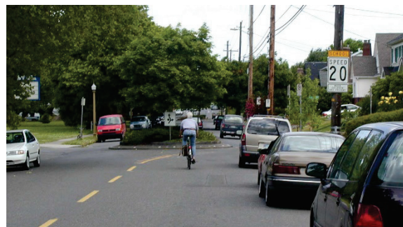
Mini circle slows traffic, creating conditions needed for shared roadway
