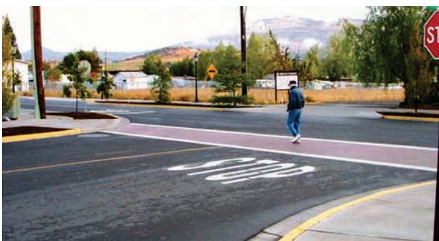
Textured crosswalk with supplemental white Markings
