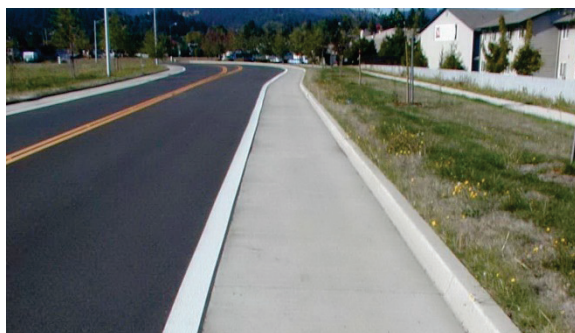
Concrete bike lane provides contrast with asphalt roadway
