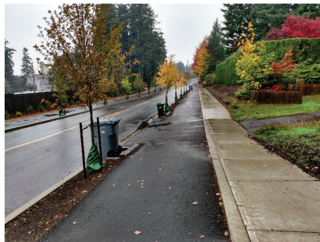
Separated bike lane with space for recycling cans in street buffer
