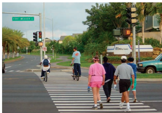
Pedestrian signal head in line with crosswalk
