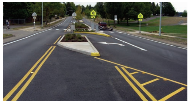
Restriped with bike lanes center turn lane and pedestrian crossing
