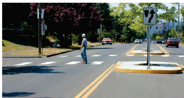
Median island provides mid-street refuge for pedestrians
