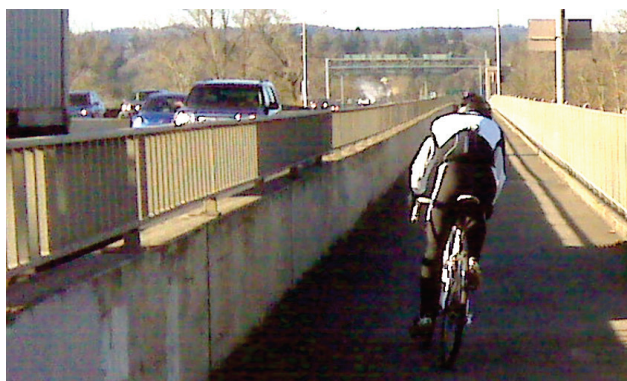
Concrete Barrier as street buffer
