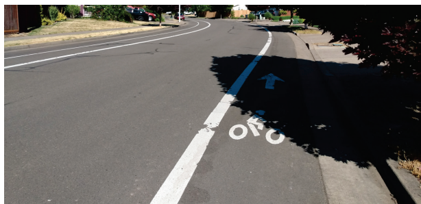
Residential Edge Lane Road (bike lanes with no center line)
