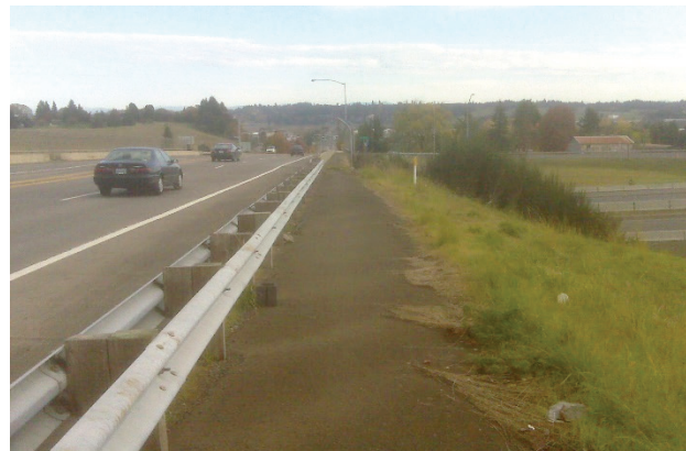
Guardrail as street buffer
