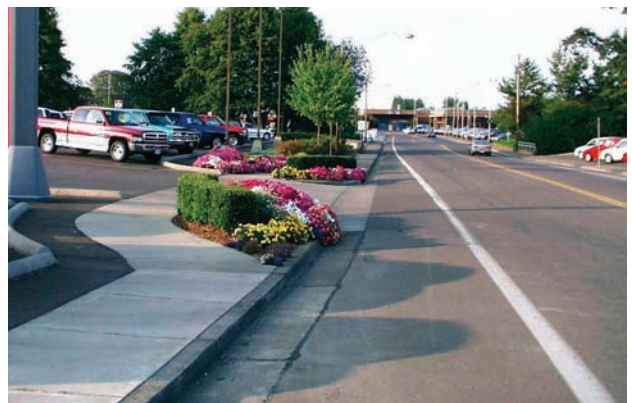
Sidewalk is kept level at driveway
