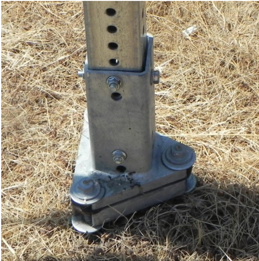
Figure 34: Slip base perforated steel square tube sign support
