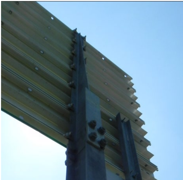
Figure 23: Extruded panel sign with fasteners
