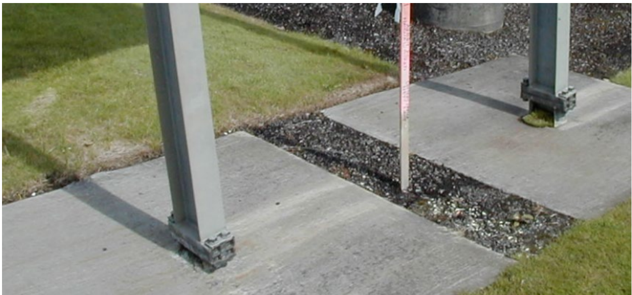
Figure 2: Multi-Post Breakaway Supports
