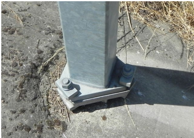
Figure 3: Standard Triangular Base Breakaway
