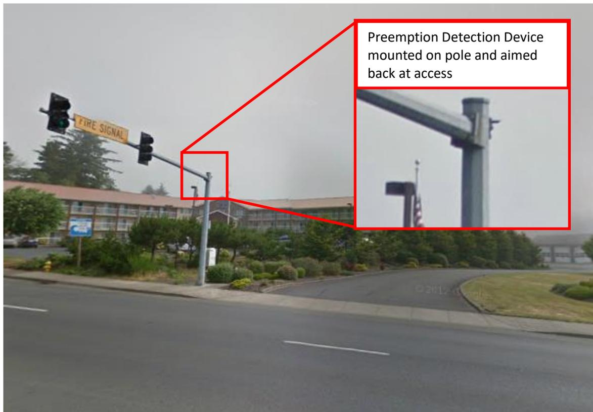
Loop detection (or any alternative vehicle detection) shall NOT be used as a preemption device. This is due to the fact that if a loop fails, the fire signal will remain preempted
