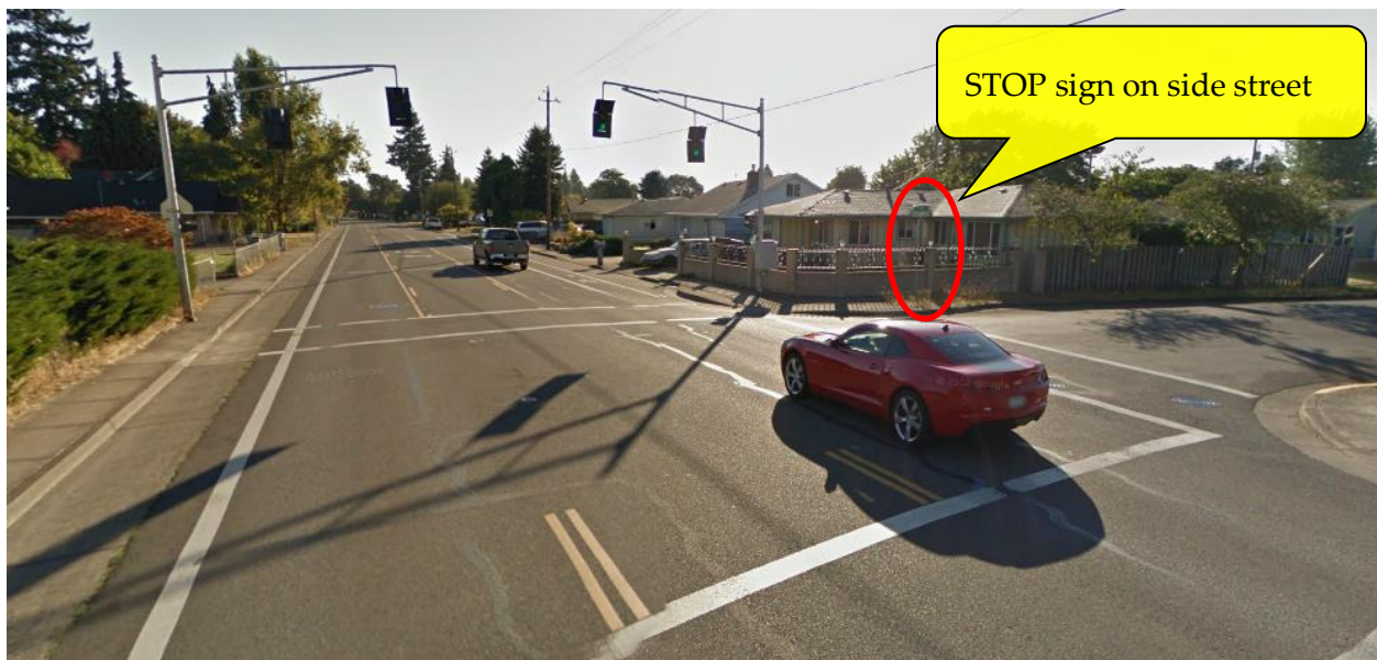
Figure 14-5 | Pedestrian Signal Installed at Intersection (Half-Signal), Prohibited
