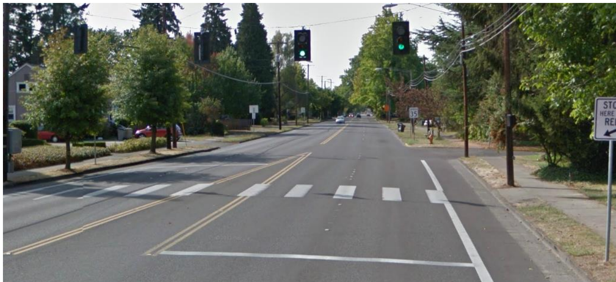
Figure 14-1 | Pedestrian Signal Installed Mid-Block, Example 1
