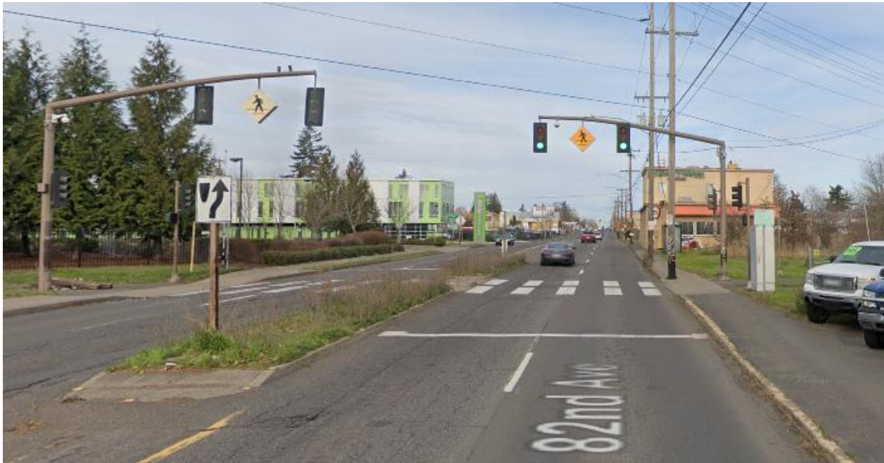
Figure 14-3 | Pedestrian Signal Installed Mid-Block, Example 3
