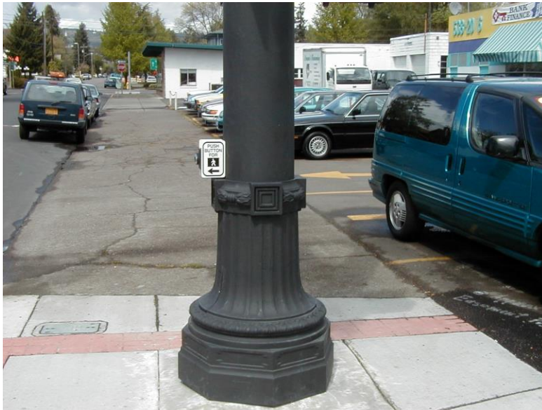
Figure 5-74 | Verification of Pushbutton Vertical Height Required (Non-Std. Equipment) – Example 2
