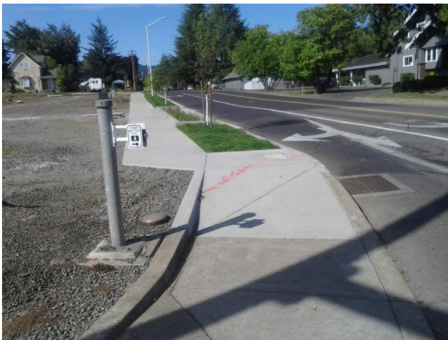
Figure 5-92 | Extension Bracket Mount Example – H-Frame
