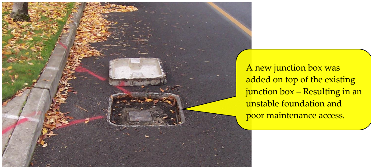
Figure 5-111 | Impacts from Raising Elevation Without Adjusting Junction Box
