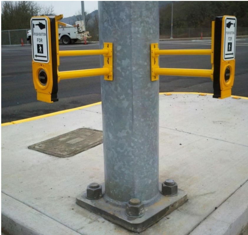
Figure 5-92 | Extension Bracket Mount Example – H-Frame
