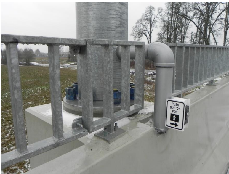
Figure 5-74 | Verification of Pushbutton Vertical Height Required (Non-Std. Equipment) – Example 2
