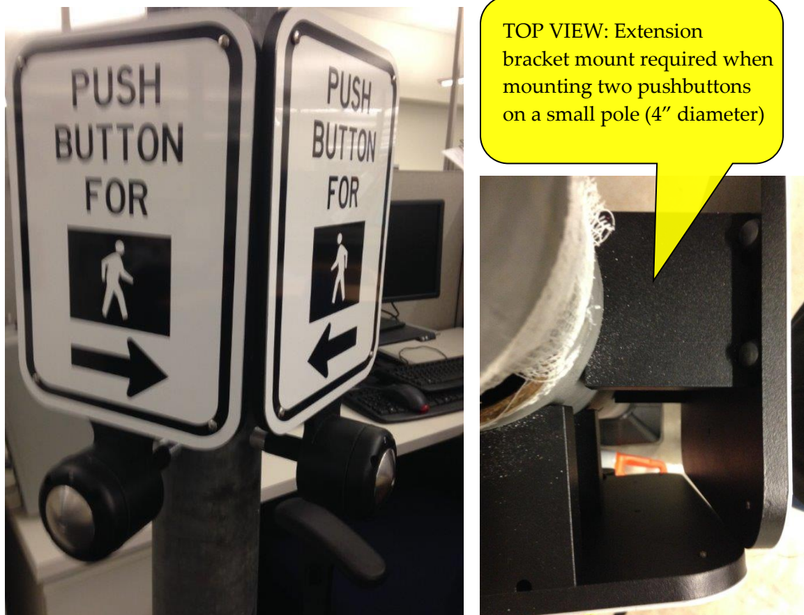
Figure 5-90 | Extension Bracket Mount for Two Pushbuttons on 4 Inch Diameter Pole
