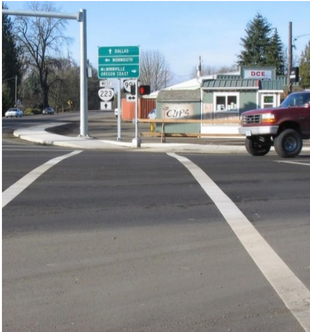
Figure 5-98 | Poor Pedestrian Signal Visibility
