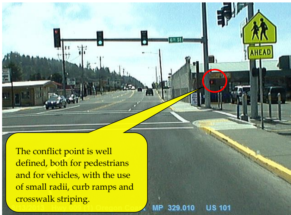
Figure 5-18 | Signalized Driveway with Small Radius and Curb Ramps (After Photo) – Use This Approach Design
