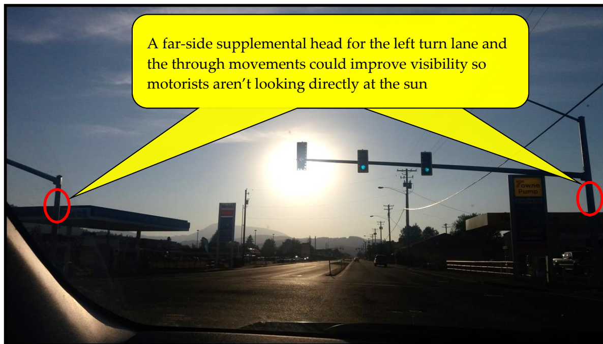
Figure 5-49 | Supplemental Signal Head Placement – Sun Glare Example
