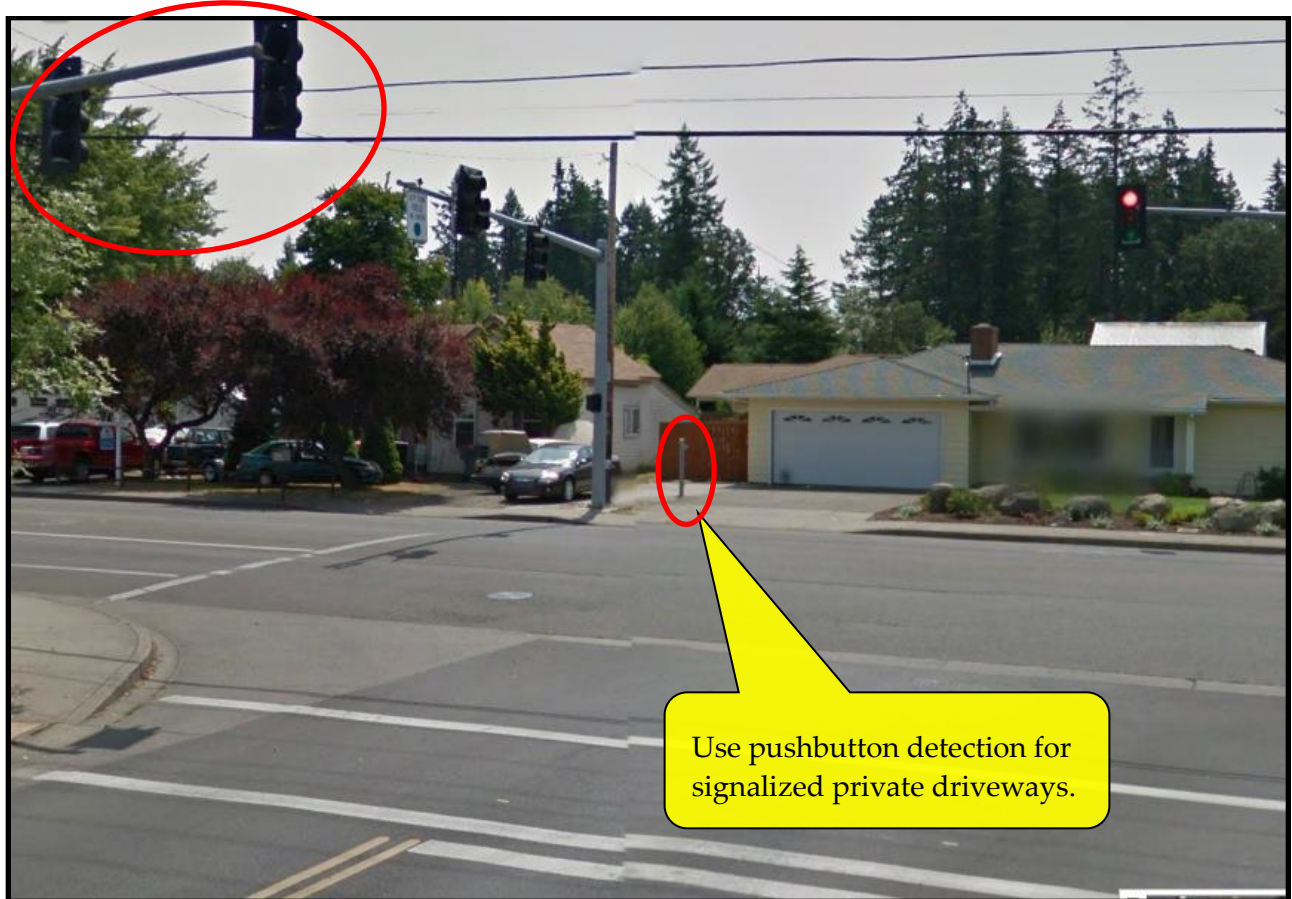
Figure 6-9 | Detection Placement Considerations: Private Driveway Signalized Approaches
