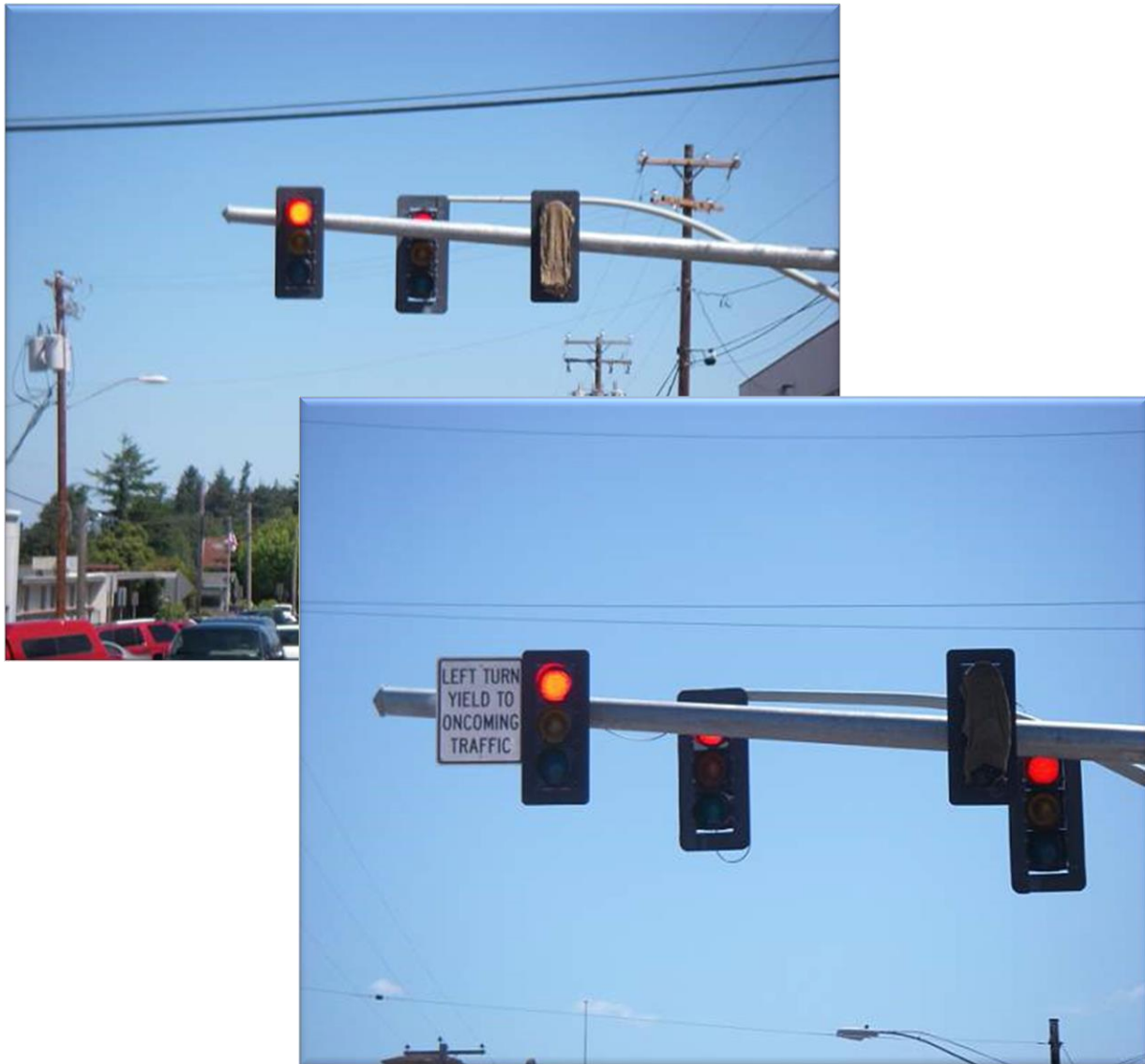
Figure 11-1 | Obstructing Signal Heads During Construction
