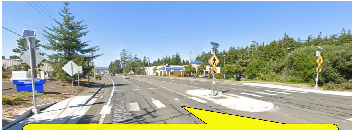
Figure 12-24 | Refuge Island Pushbutton Recommended: Total Number of Lanes Crossed by the Pedestrian is Greater Than Four
