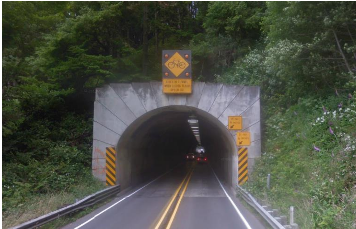
Figure 12-11 | Actuated Warning Beacon – Tunnel, Example 2
