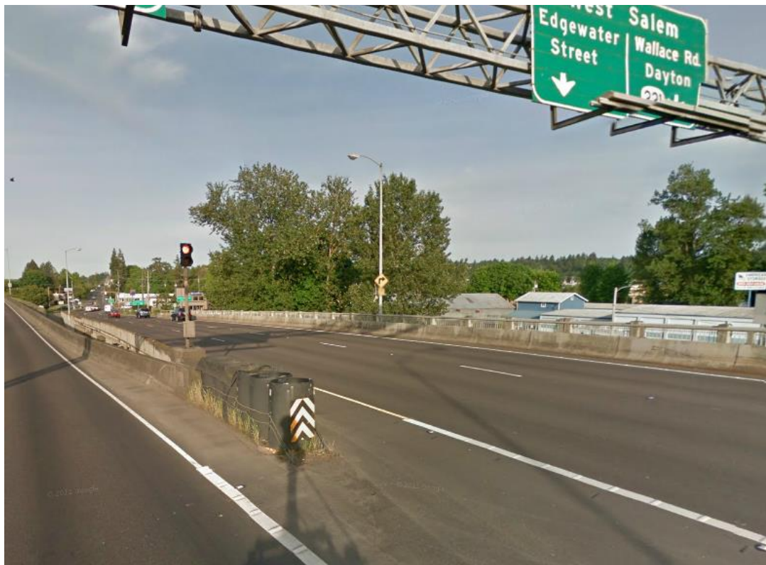
Figure 12-4 | Warning Beacon for an Obstruction, Example 1
