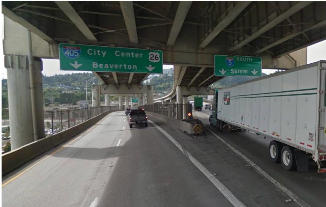
Figure 12-5 | Warning Beacon for an Obstruction, Example 2
