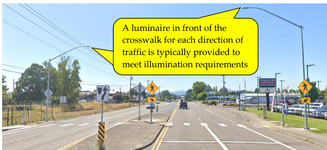
Figure 12-28 | RRFB Illumination Example
