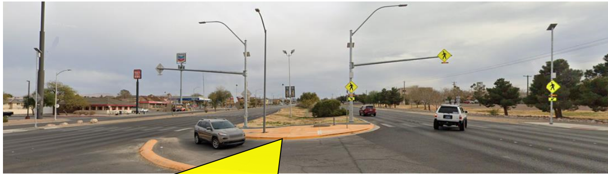
Figure 12-25 | Refuge Island Pushbutton Recommended: Wide Refuge Island
