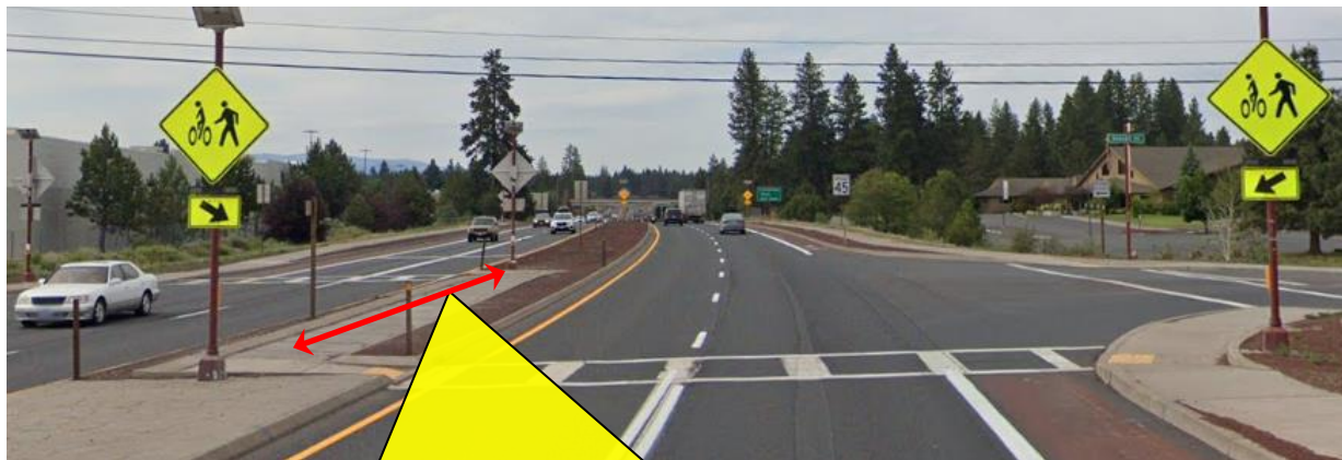
Figure 12-26 | Refuge Island Pushbutton Recommended: Staggered Crosswalks Requiring Pedestrians to Walk a Significant Distance
