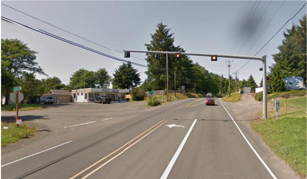
Figure 12-33 | Intersection Control Beacon, Mast Arm, Example 2
