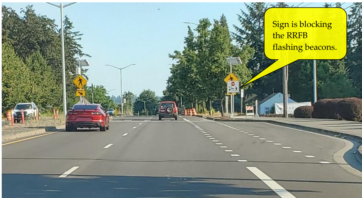
Figure 12-2 | Sight Distance Considerations – Closely Spaced Sign Can Obstruct the Flashing Beacon
