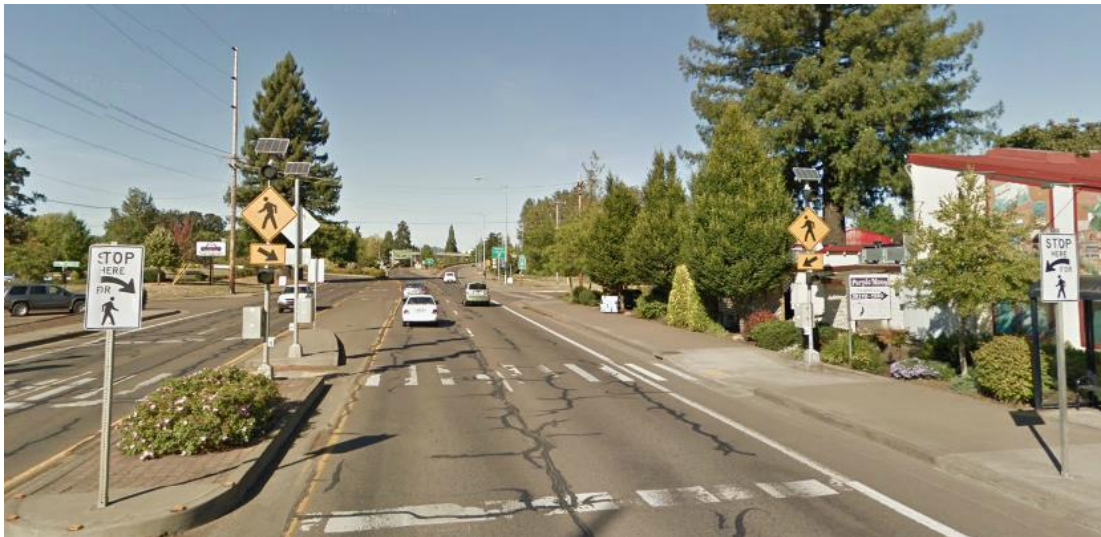
Figure 12-15 | Warning Beacon for a Warning Sign, Actuated Operation, Ground Mounted
