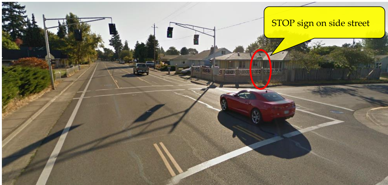
Figure 14-5 | Pedestrian Signal Installed at Intersection (Half-Signal), Prohibited
