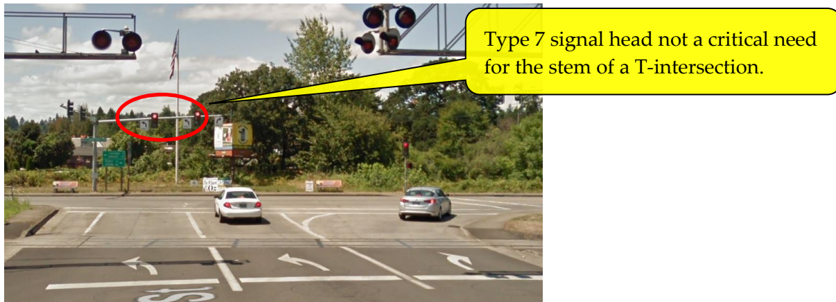
Figure 16-32 | Permissive Only Left Turn (No Oncoming Traffic) – Type 7 Signal Head Not Critical for Proper Preemption Operation
