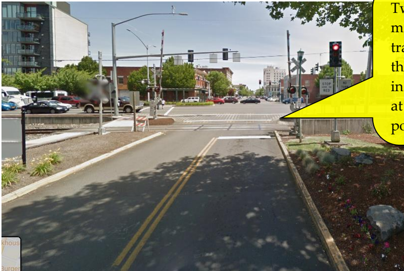
Figure 16-17 | Crosswalk Prior to Railroad Crossing Example 2
