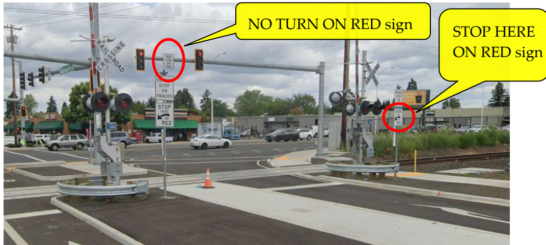
Figure 16-25 | STOP HERE ON RED sign example 1
