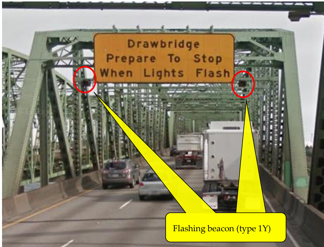
Figure 24-16 | Columbia River NB: 2 st Warning Device
