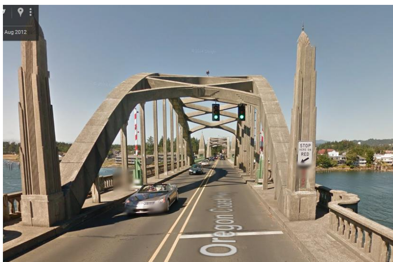
Figure 24-11 | Signal Heads and Sign Custom Mounted on Bridge Structure
