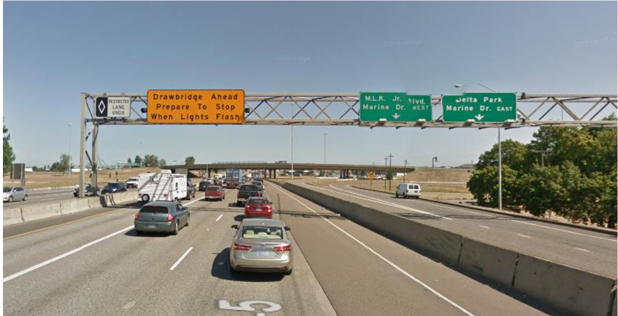
Figure 24-15 | Columbia River NB: 1 st Warning Device
