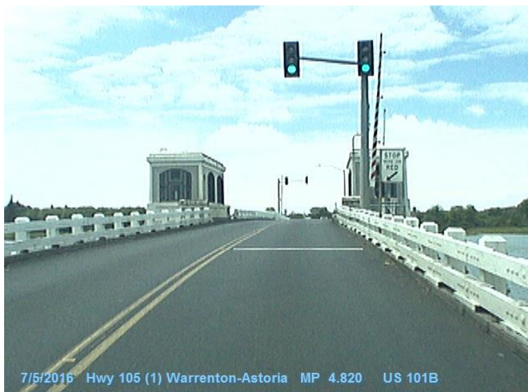
Figure 24-11 | Signal Heads and Sign Custom Mounted on Bridge Structure
