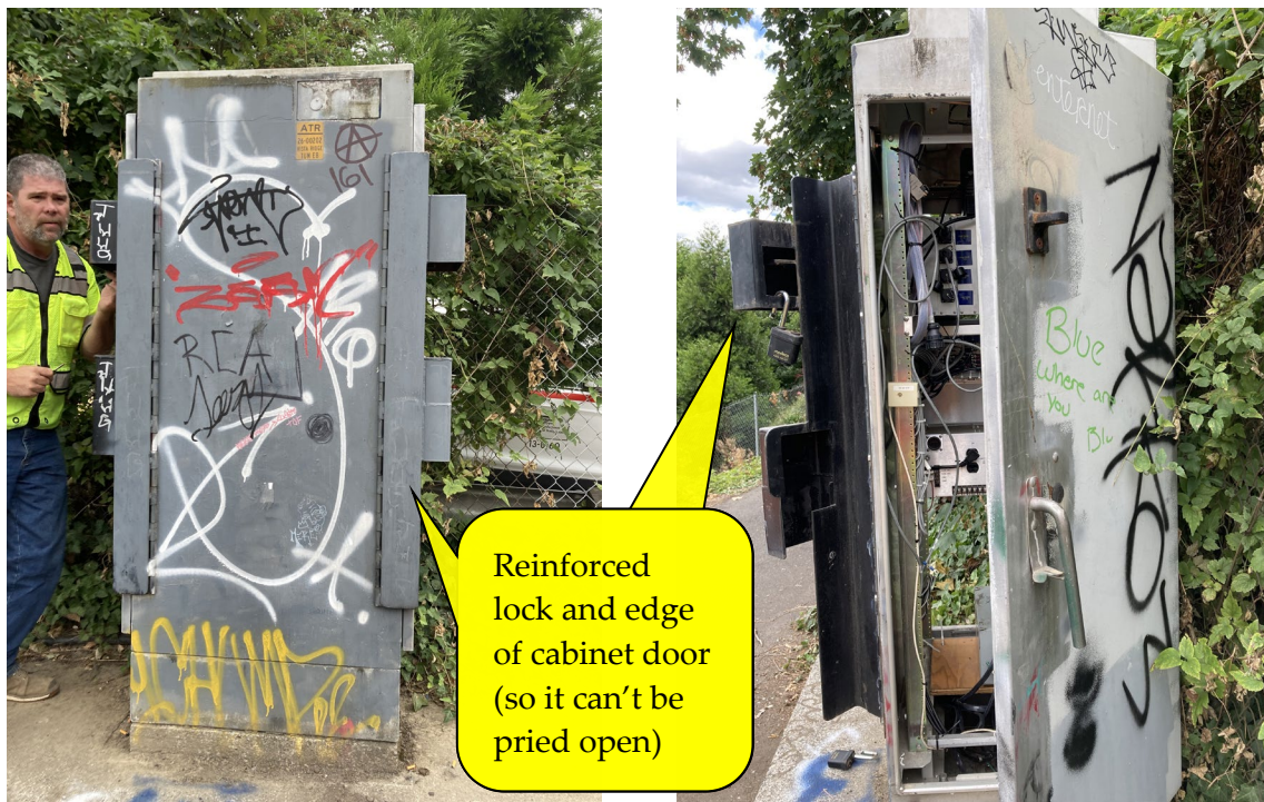
Figure 25-22 | Anti-Vandalism Treatment – Custom Locking Mechanism
