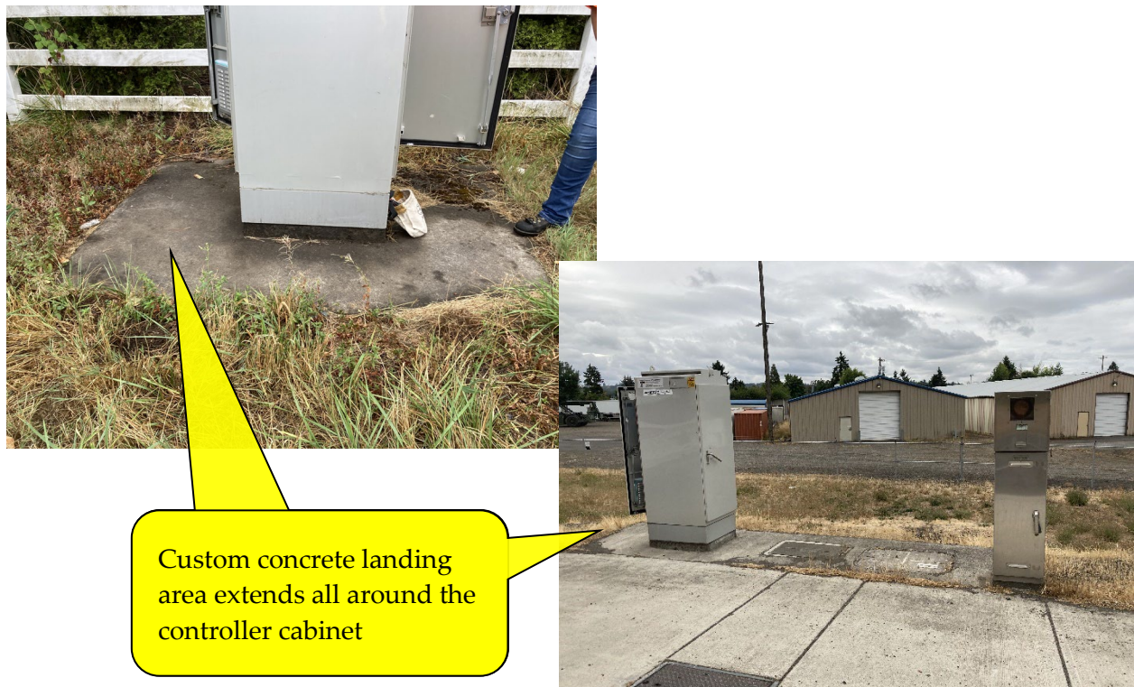
Figure 25-17 | Custom Controller Cabinet Landing Area Examples
