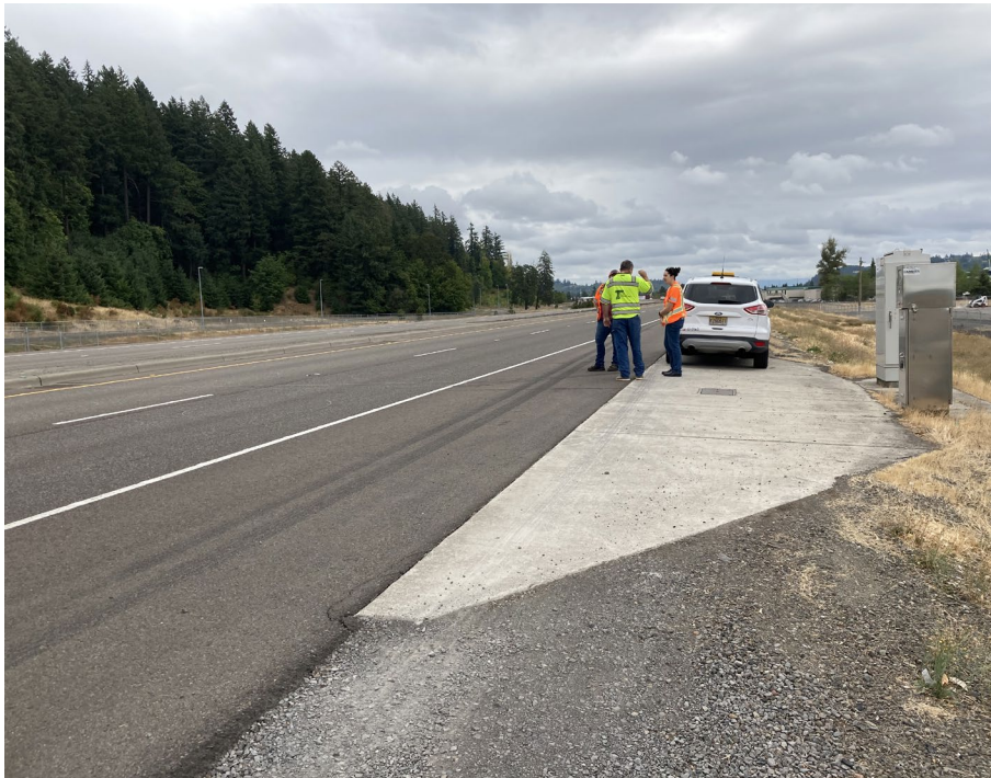
Figure 25-20 | ATR Site Maintenance Pad Example
