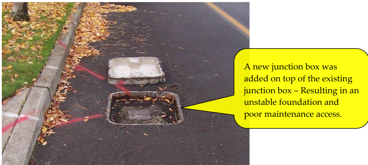
Figure 5-115 | Impacts from Raising Elevation Without Adjusting Junction Box
