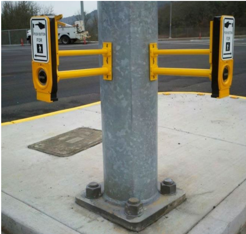
Figure 5-95 | Extension Bracket Mount Example – H-Frame
