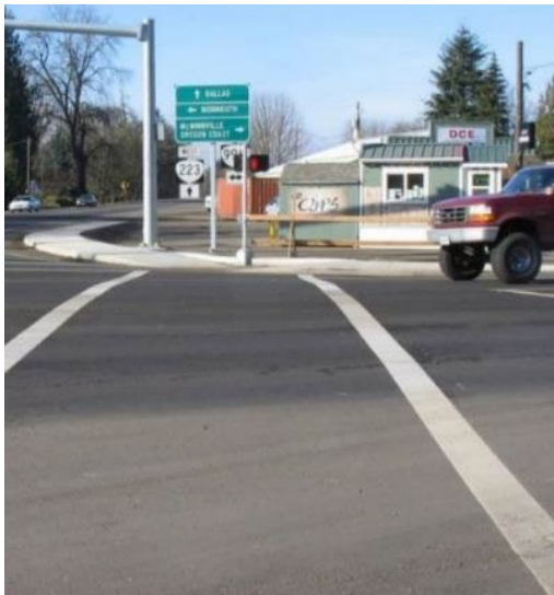
Figure 5-101 | Poor Pedestrian Signal Visibility
