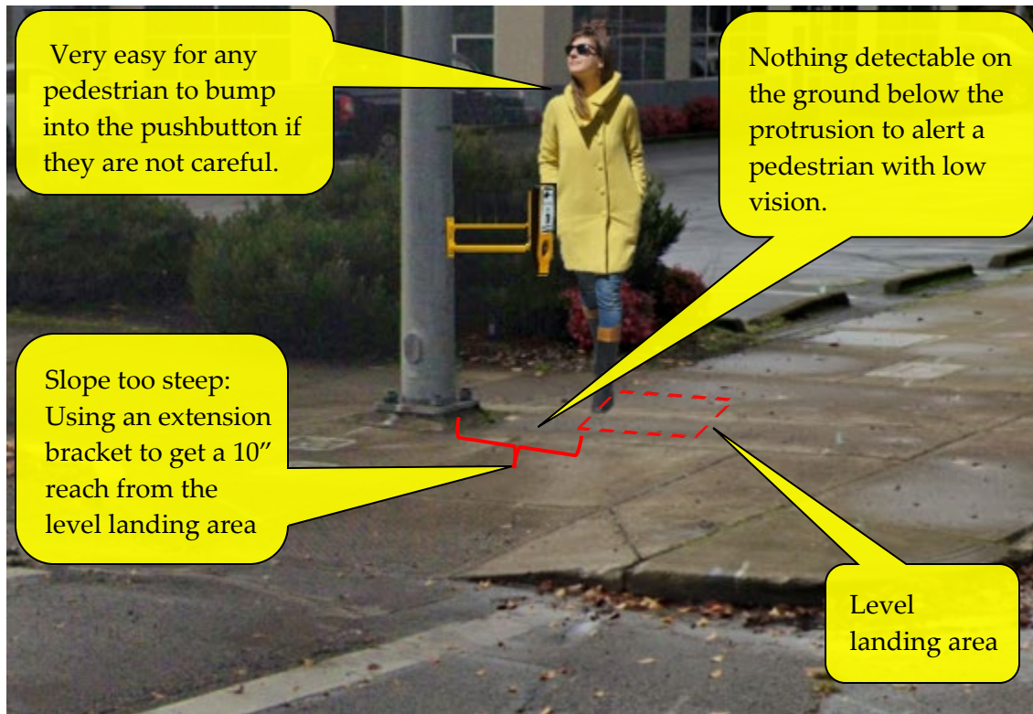
Figure 5-96 | Extension Bracket Mount Photoshop Example – Extending More Than 4 Inches into the Pedestrian Circulation Path
