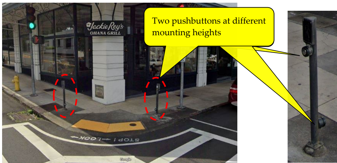
Figure 5-97 | Deviation to Vertical Reach Example
