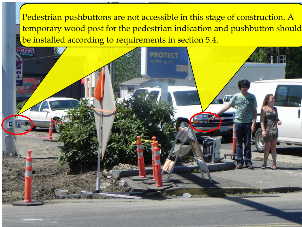
Figure 11-8 | Pedestrian Pushbutton Access – Example 1
