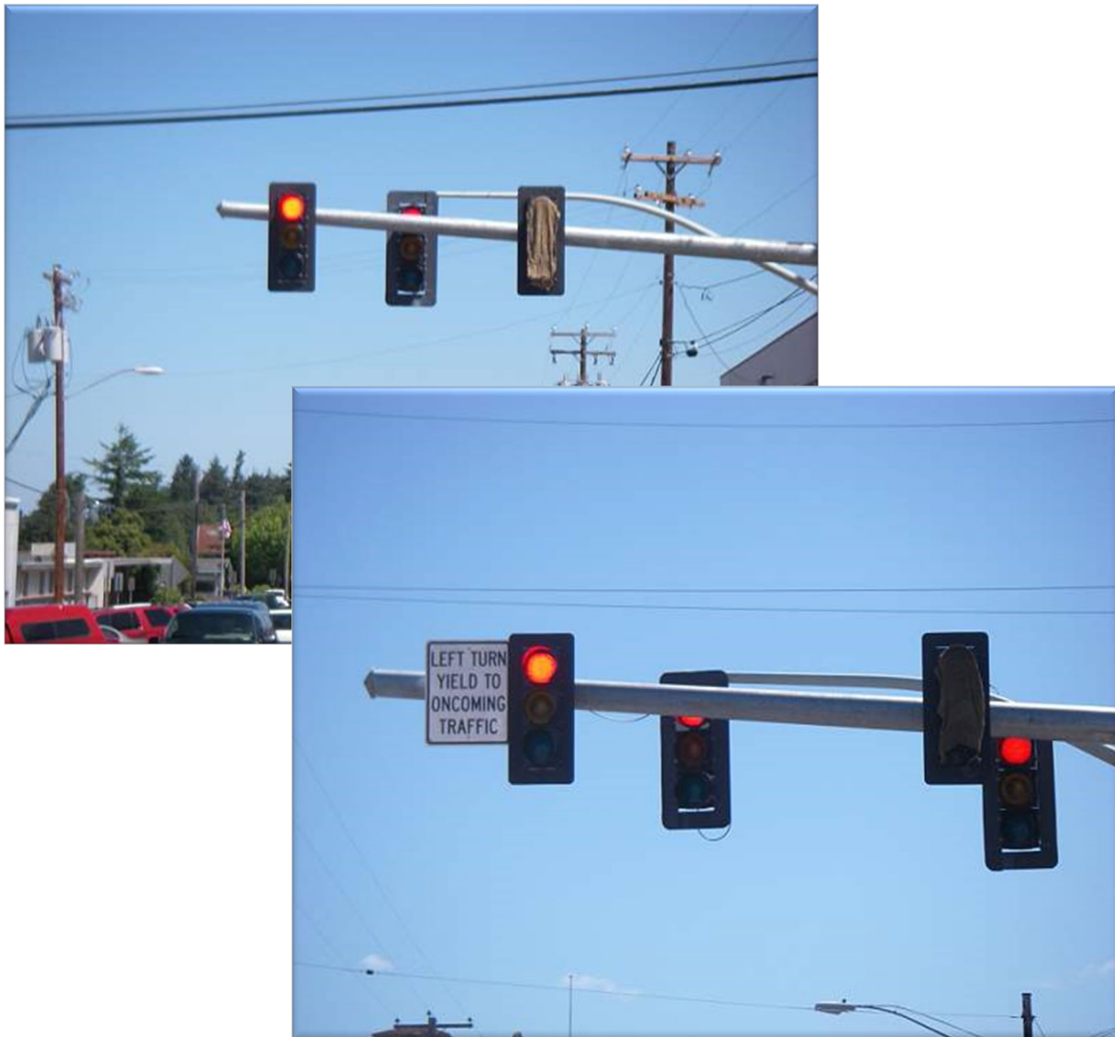
Figure 11-1 | Obstructing Signal Heads During Construction
