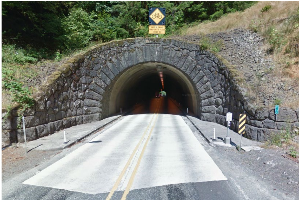
Figure 12-11 | Actuated Warning Beacon – Tunnel, Example 2
