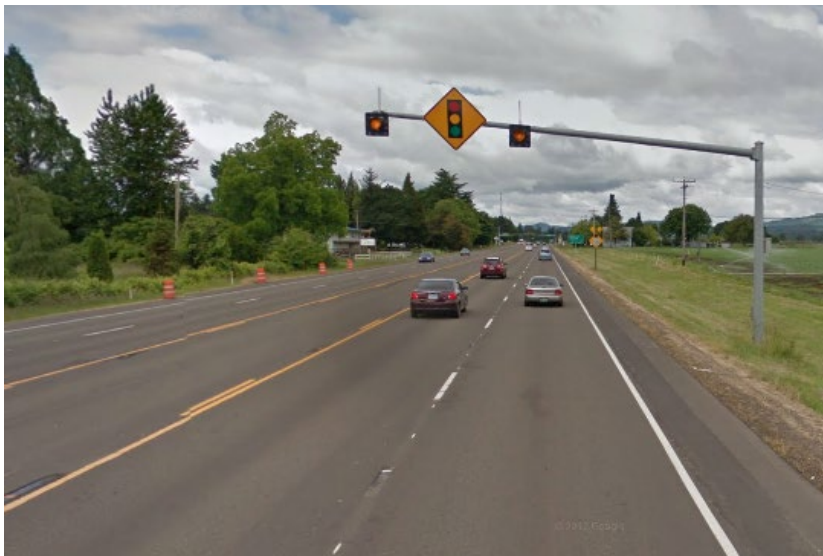
Figure 12-7 | Warning Beacon for a Warning Sign, Overhead
