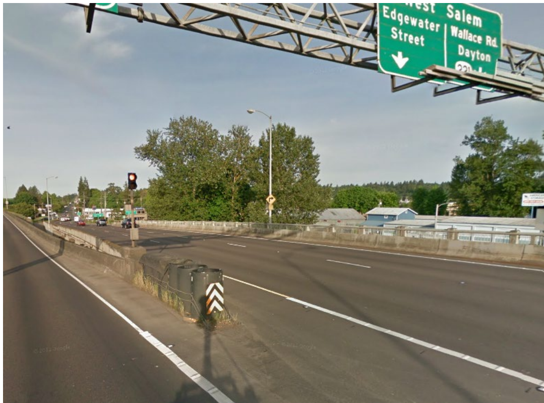
Figure 12-4 | Warning Beacon for an Obstruction, Example 1
