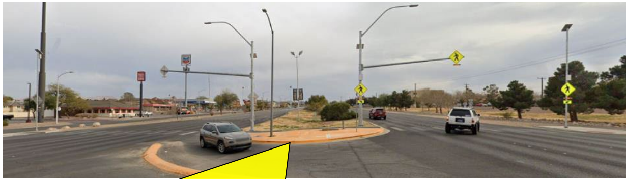
Figure 12-25 | Refuge Island Pushbutton Recommended: Wide Refuge Island
