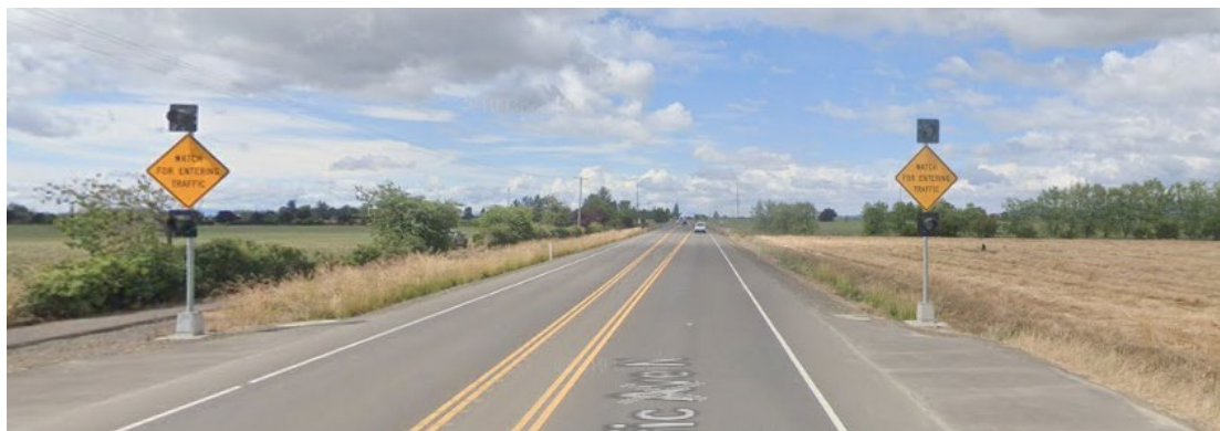
Figure 12-17 | TRAWS Location and Placement Example
