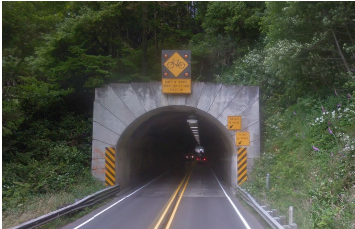
Figure 12-11 | Actuated Warning Beacon – Tunnel, Example 2
