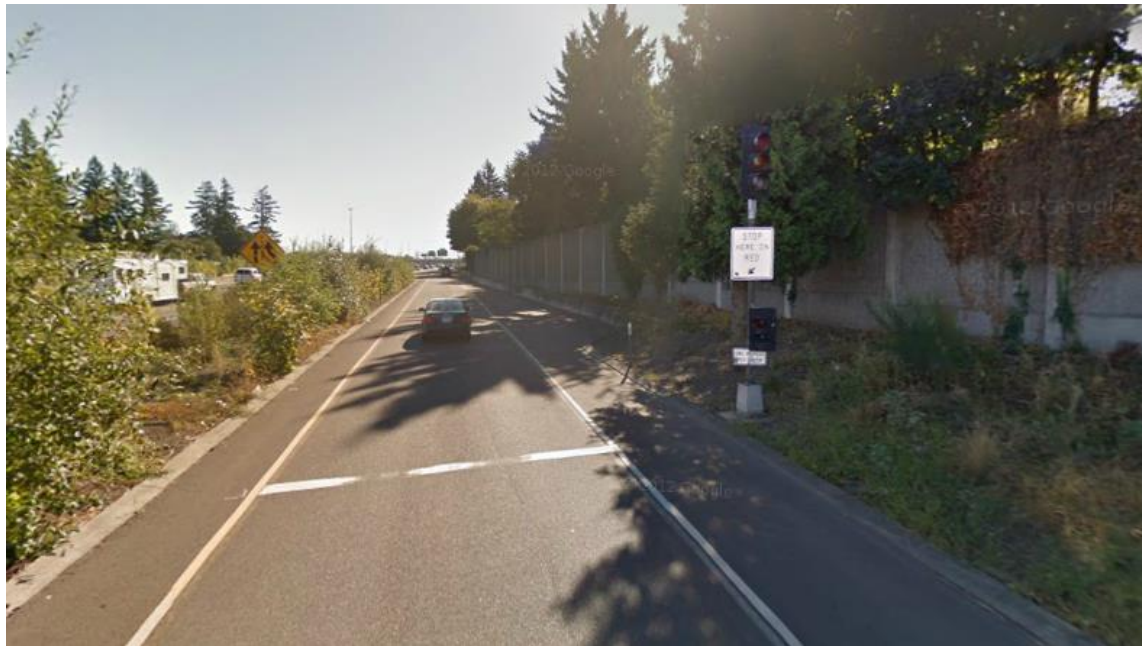
Figure 13-6 |Ramp Meter Signal Assembly Example – Controlling Two Lanes of Traffic
