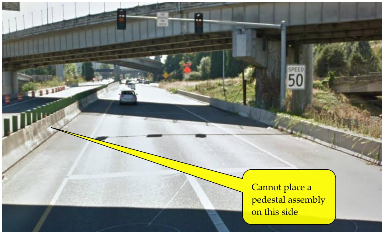
Figure 13-3 | Physical Constraints (Barrier on Left Side) - Requires Overhead Mount
