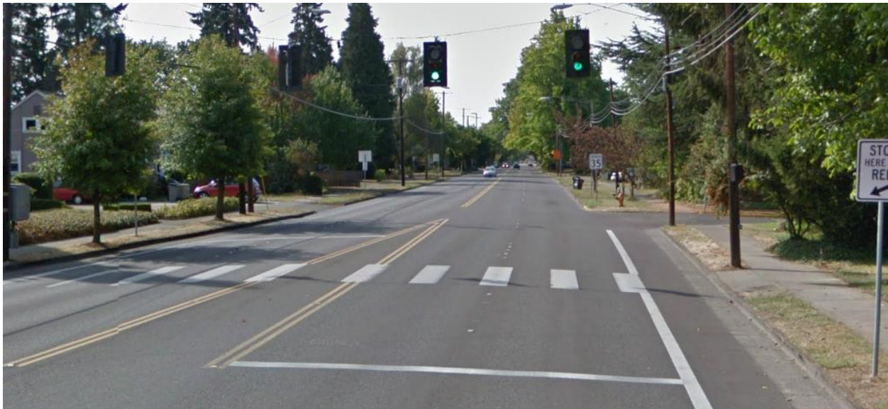
Figure 14-1 | Pedestrian Signal Installed Mid-Block, Example 1
