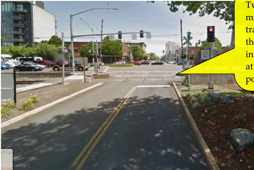
Figure 16-17 | Crosswalk Prior to Railroad Crossing Example 2
