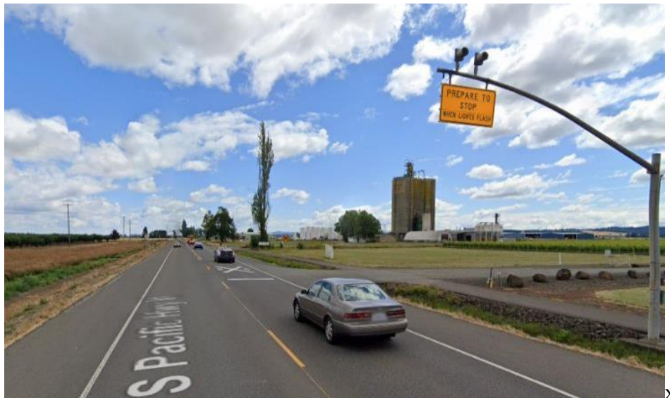
Figure 16-37 | Example 2 of Rail Controller Cabinet Activated Traffic Control Device
