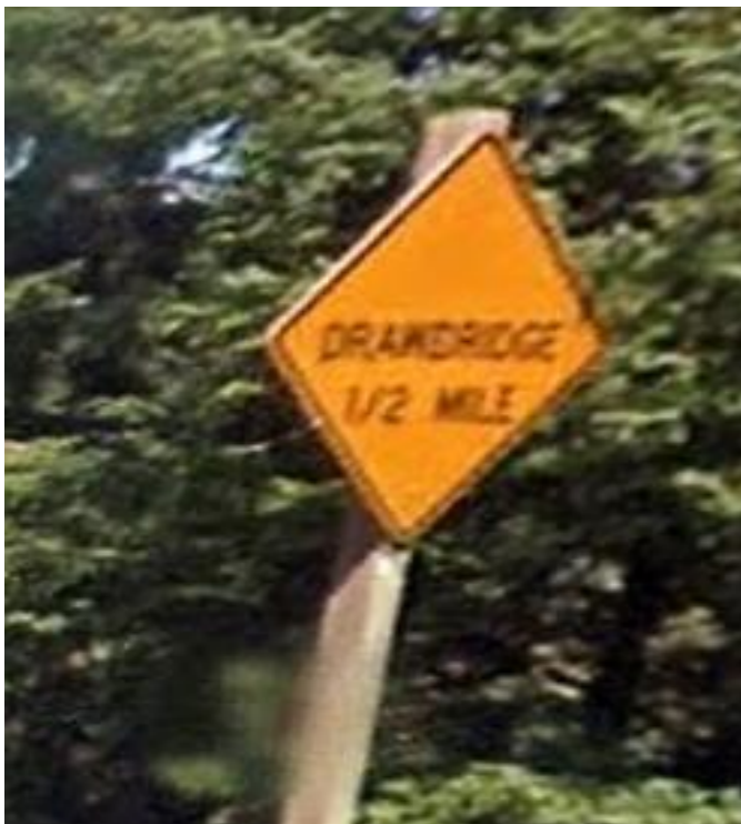
Figure 24-7 | Non-Compliant Existing TCD: Outdated Signs, Example 2
