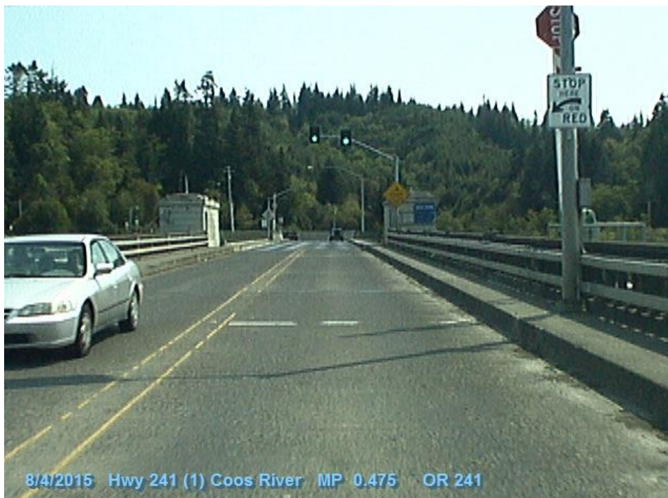
Figure 24-3 | Non-Compliant Existing TCD: Mounting a STOP Sign to the Warning Gate
