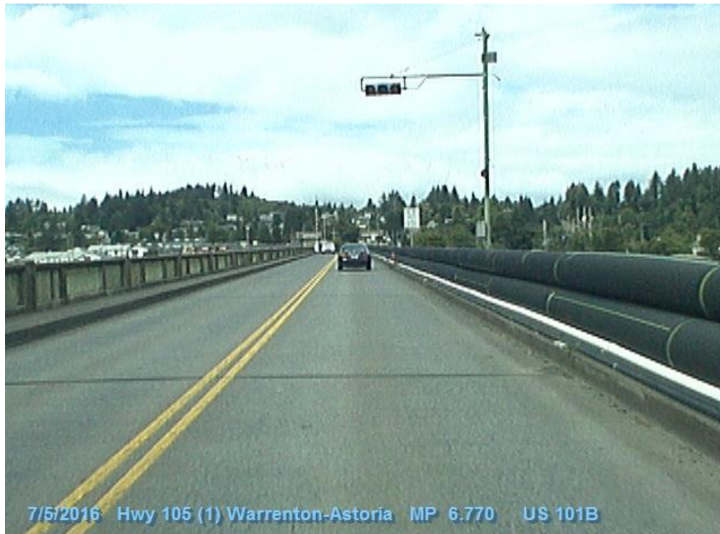
Figure 24-5 | Non-Compliant Existing TCD: Single Advance Signal Head, Example 2
