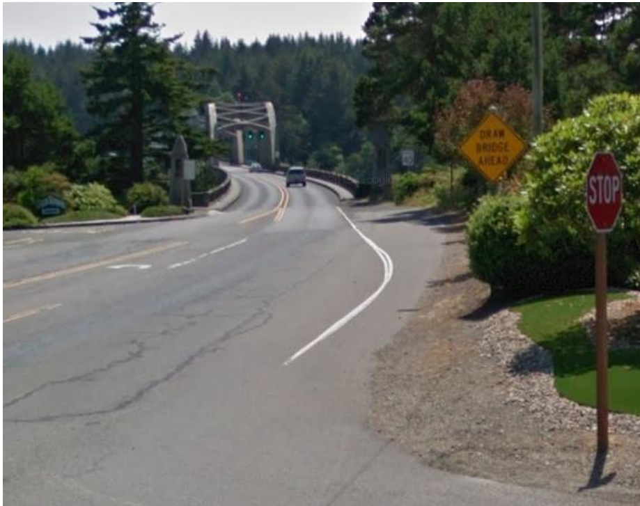
Figure 24-7 | Non-Compliant Existing TCD: Outdated Signs, Example 2
