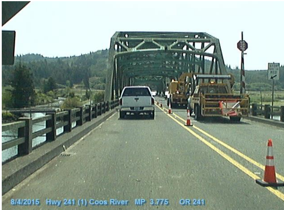
Figure 24-3 | Non-Compliant Existing TCD: Mounting a STOP Sign to the Warning Gate
