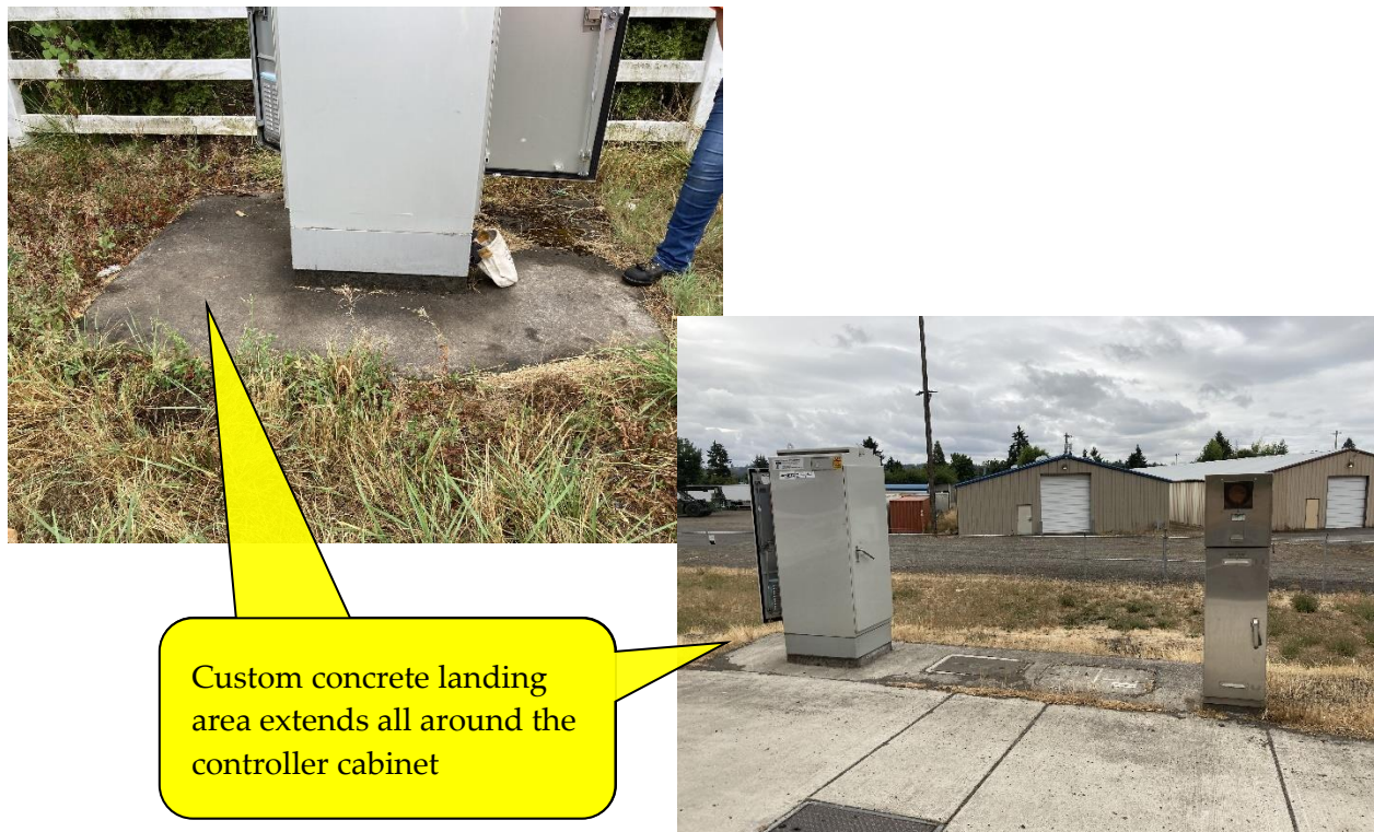
Figure 25-17 | Custom Controller Cabinet Landing Area Examples
