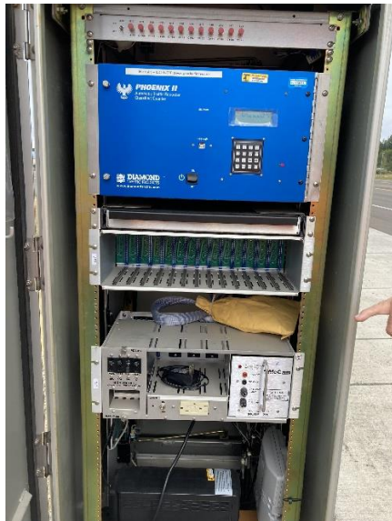
Figure 25-19 | Two Phoenix II Controllers – Accommodates 32 Loop Detectors and 16 Piezos
