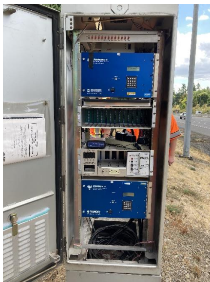
Figure 25-19 | Two Phoenix II Controllers – Accommodates 32 Loop Detectors and 16 Piezos
