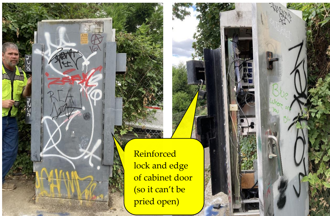
Figure 25-22 | Anti-Vandalism Treatment – Custom Locking Mechanism
