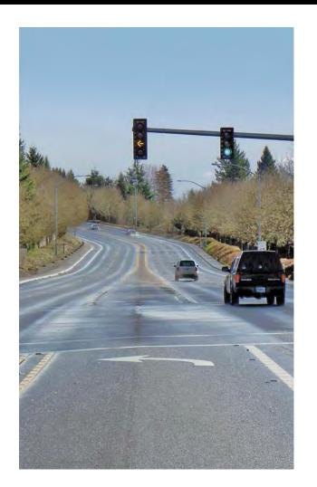
**Safer** – The Federal Highway Administration has found that up to 20% fewer crashes occur with FYA than the traditional signal. Drivers have less confusion and make fewer mistakes when turning with FYA.
