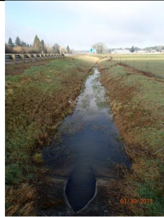
Example of photo 7 Facility outlet/outfall (outlet channel from pond drains to nearby creek)
