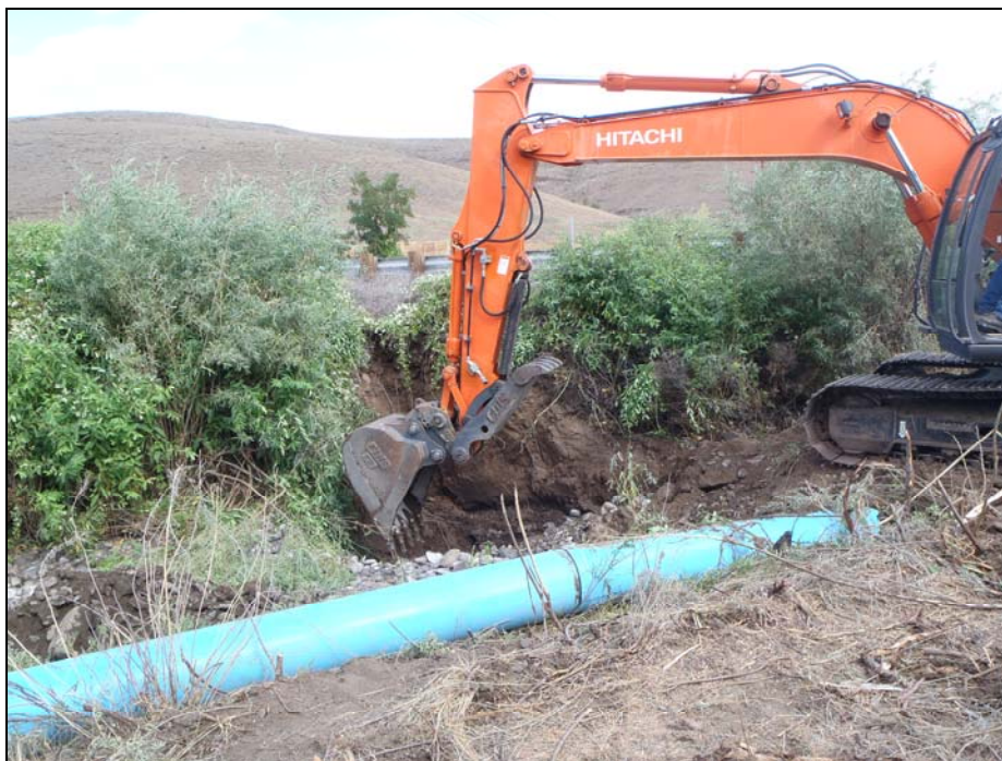
Photograph 1: View of excavation for barb, facing 350°. 8/2/13 (13-037:6)
