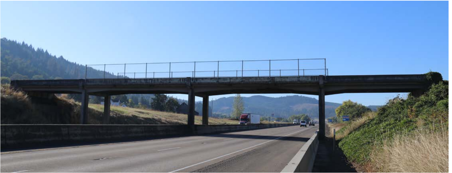
Photo 1: I-5 MP149.39 Equipment Overpass Bridge (Bridge #07643), looking South (taken 10/4/17 by Kenny Gunn)
