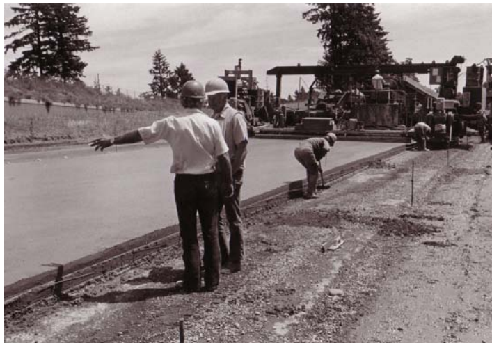
Figure 13. Continuous concrete paving, c. 1963 (Source: ODOT GF).
