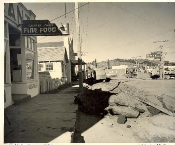
Figure 4 — Historic photo of road and sidewalk repairs, Gold Beach, OR (ODOT, 1949). In 17 years, pedestrian-designated space was established and roads were asphalt-paved.
