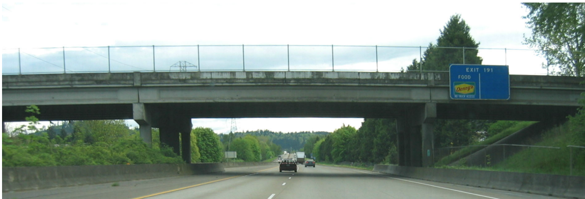
Figure 1.19. Typical Pre-cast I-Beam Overpass, Interstate 5, Lane County, OR Source: Author Photograph, May 2002
