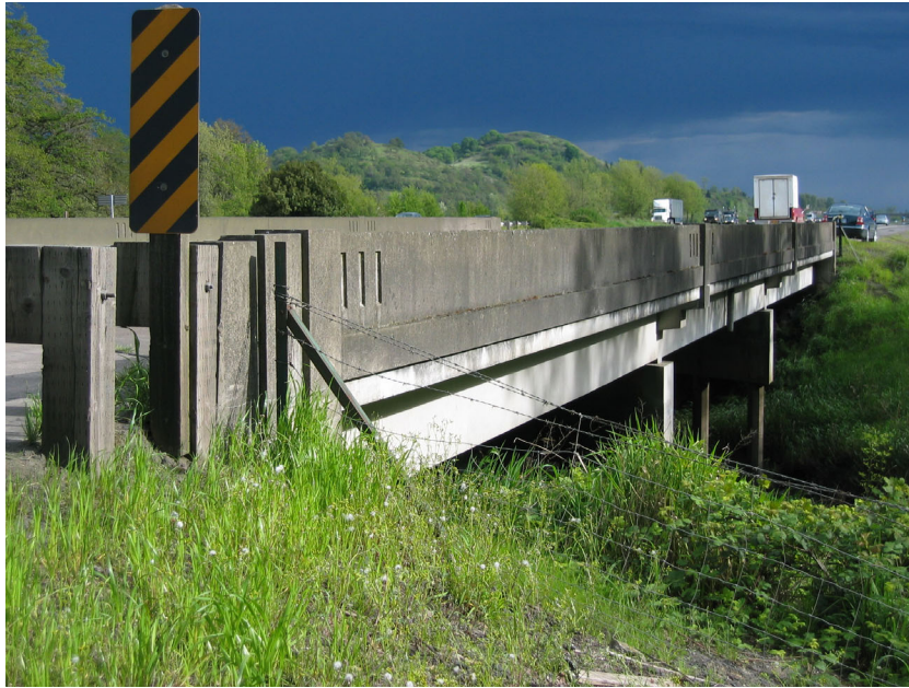
Figure 2.8. Type A/B Bridge Replacement Rail Isaac Constant Bridge, Central Point, Oregon Source: Author Photograph, November 2002
