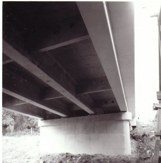
Figure 2.29. Flat Panel Concrete Pier, Pudding River and Butte Creek Overflow, 1970 Source: ODOT Archive
