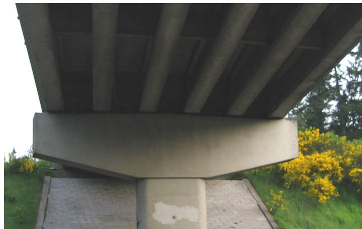
Figure 2.30. Various Monolithic Concrete Bridge Pier Designs Interstate-5 Examples Source: Author Photographs, May 2002
