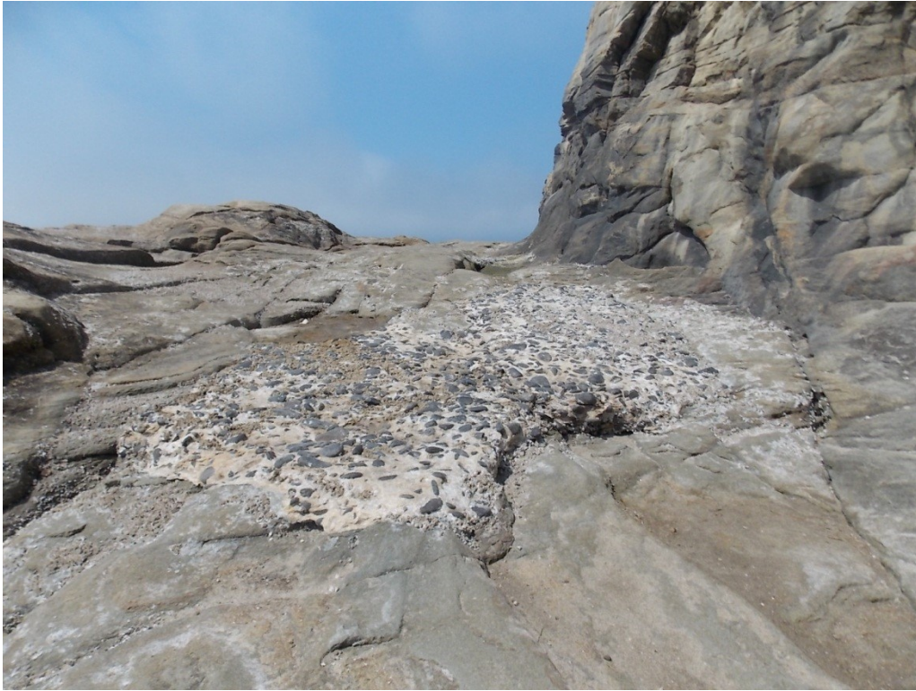
Figure 5. View of the remaining macadam paving around Hug Point
