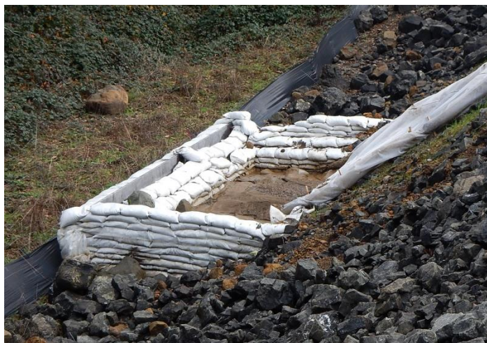
Figure 2-13 Sediment Trap & Energy Dissipater W/ Level Spreader
