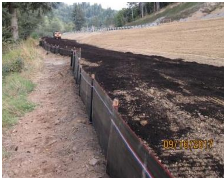
Figure 3-27 Sediment fence is trenched in correctly
