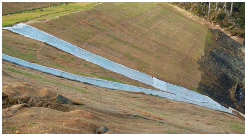
Figure 3-13 Plastic sheeting runoff control on slope matting
