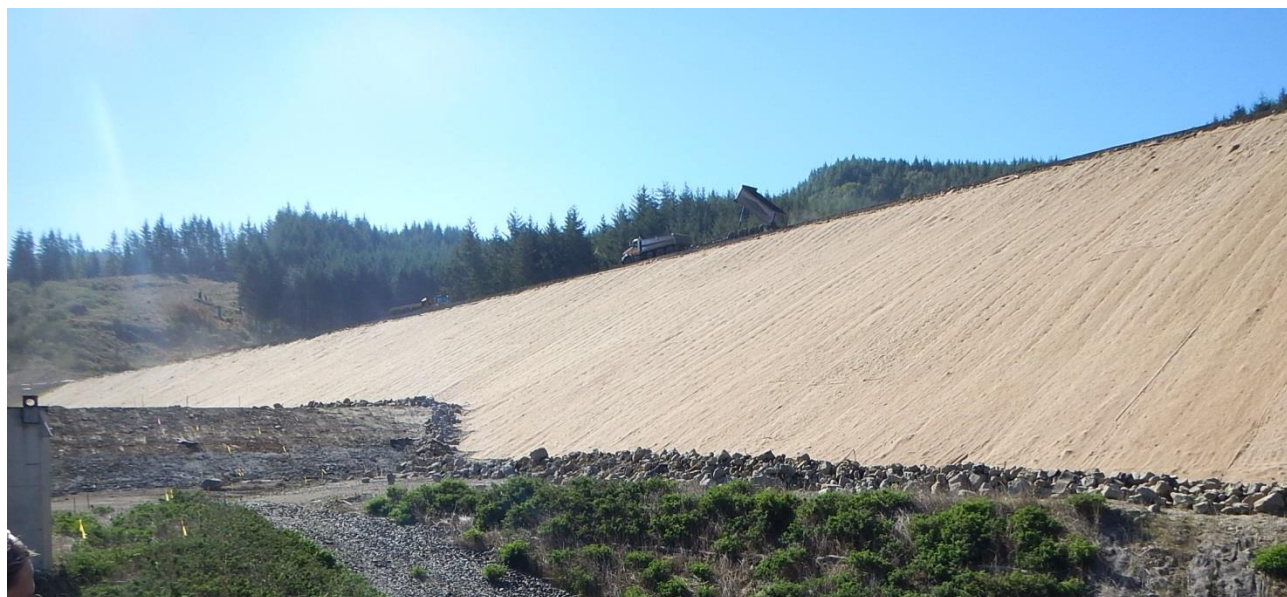
Figure 3-10 fully biodegradable slope protection matting
