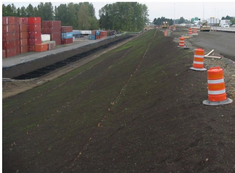
Figure 3-12 Compost blankets provides erosion prevention
