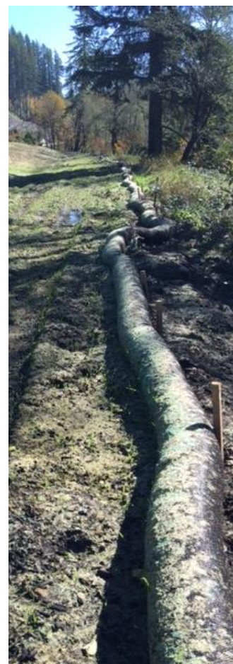
Figure 3-23 Compost Sock – Sediment Barrier Type 8
