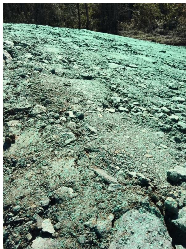
Figure 3-7 Thin hydromulch application
