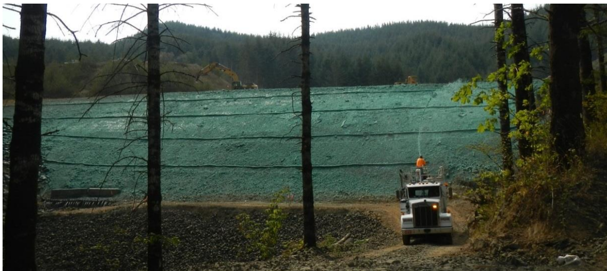
Figure 3-4 Seeding & mulch applied with Hydroseeder
