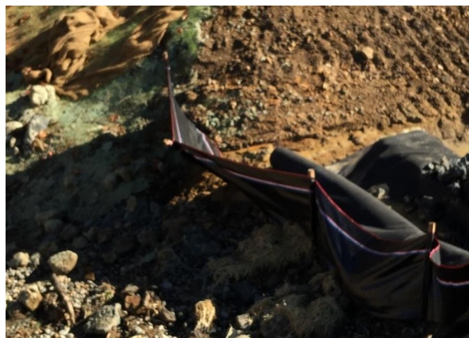
Figure 3-30 Sediment fence not embedded in ground
