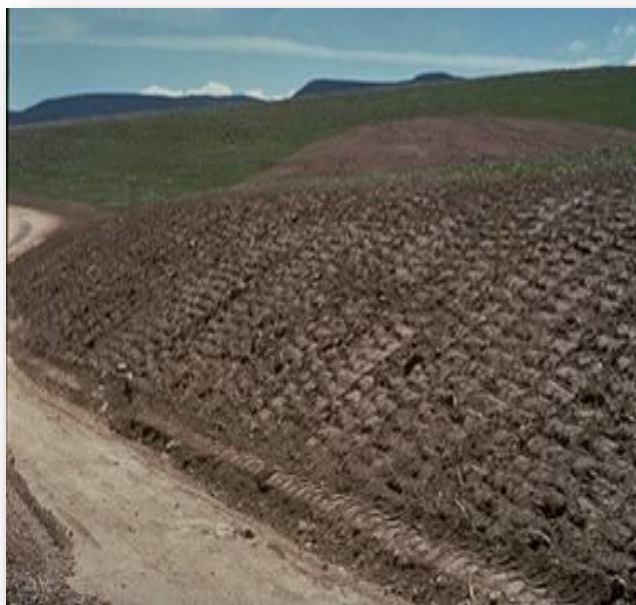
Figure 3-3 Roughened Soil Surface
