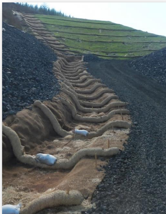
Figure 2-12 Stabilized Channel
