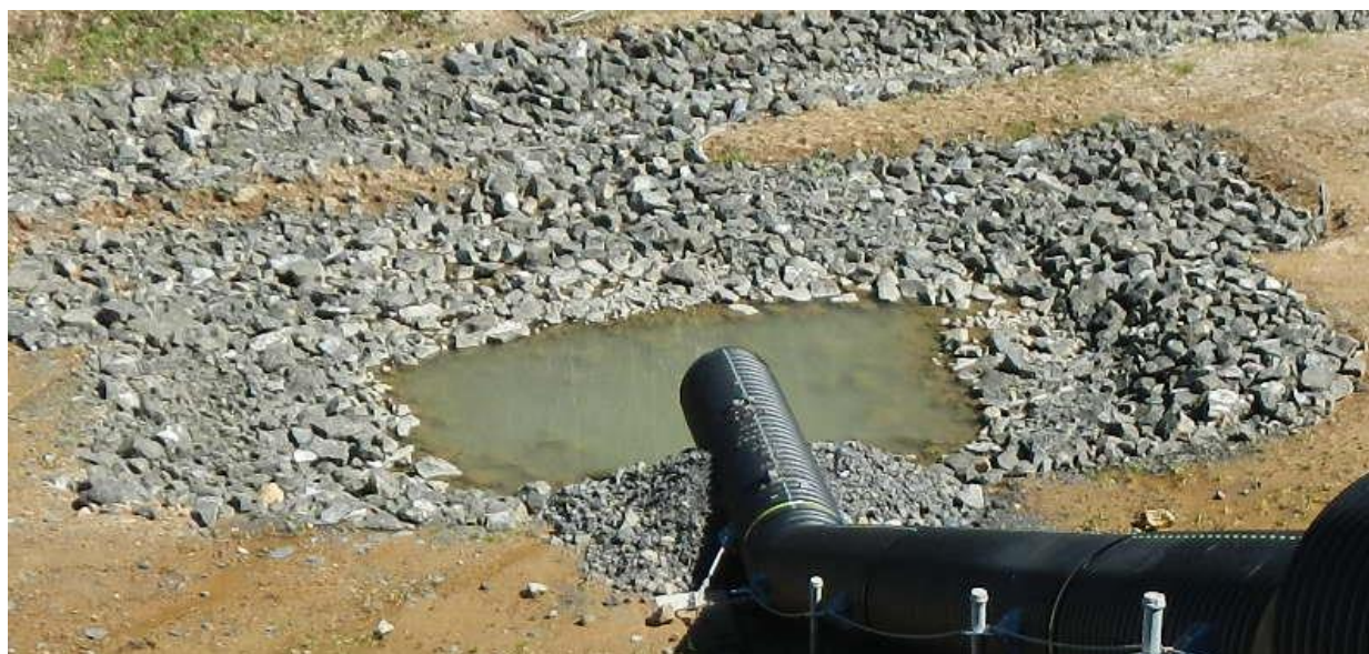
Figure 3-16 Energy Dissipater (permanent installation)
