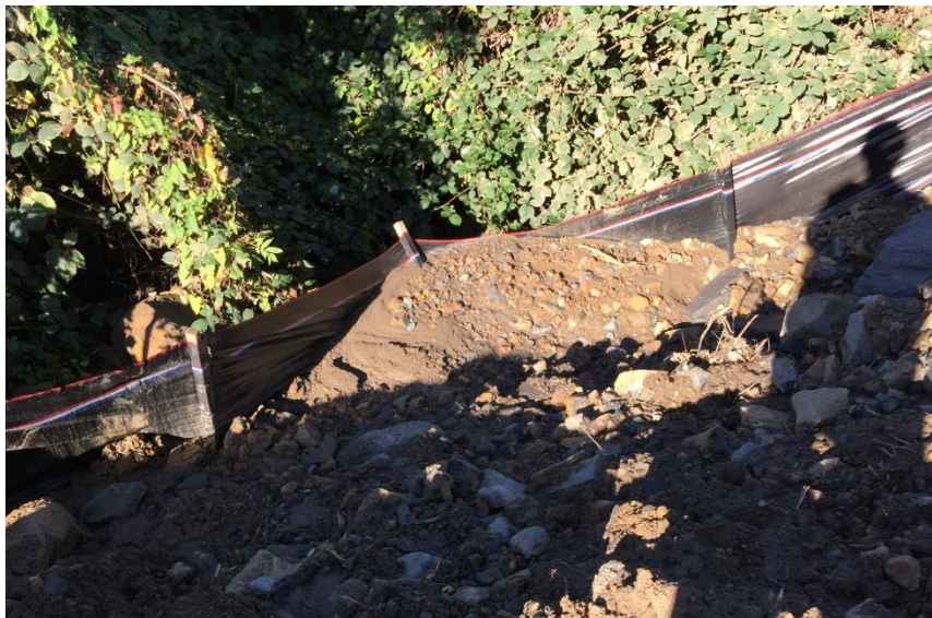
Figure 3-29 Sediment fence maintenance failure
