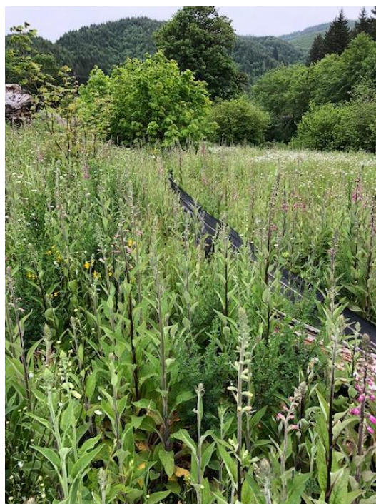
Figure 3-28 Sediment fence should be removed once vegetation is established
