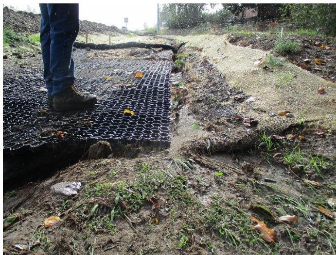
Figure 2-7 Erosion control failure at water quality facility
