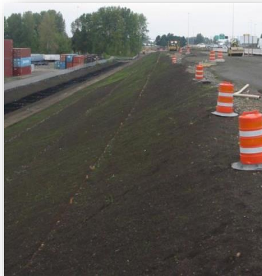
Figure 2-9 Compost blankets provides erosion prevention
