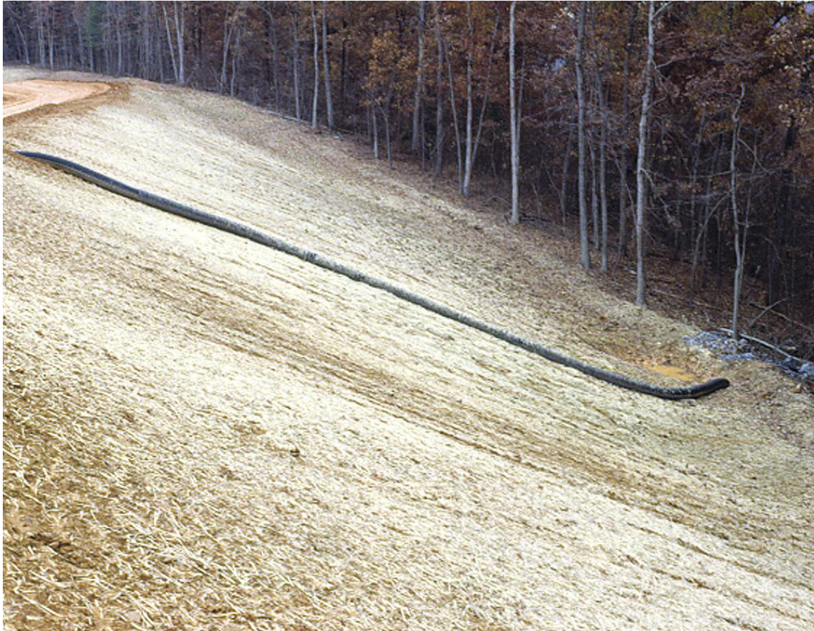
Figure 3-14 Temporary Slope Drains
