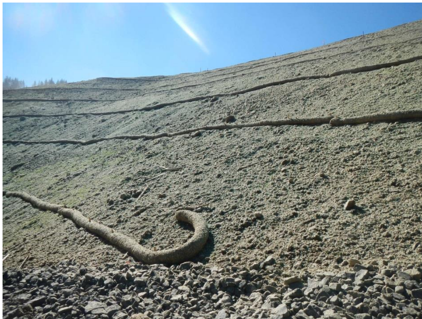
Figure 3-22 Fiber Rolls (Wattles) – Sediment Barrier Type 3
