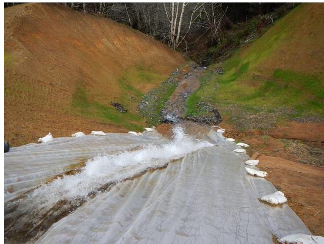
Figure 3-15 Plastic sheeting used as Temporary Slope Drains
