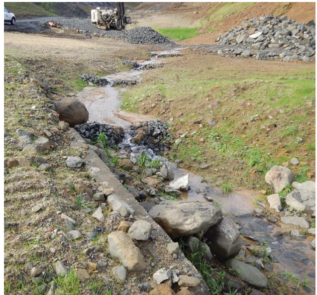
Figure 2-11 Check Dams slow runoff velocity
