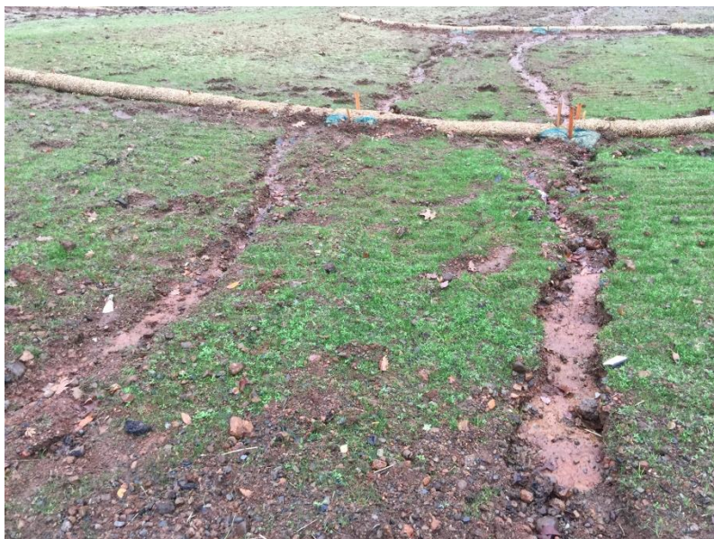
Figure 2-4 Rills on a Slope
